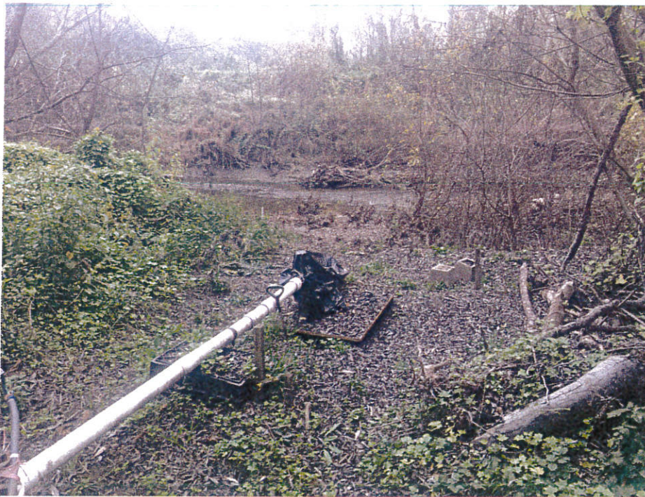
Photo # 3 point of diversion
