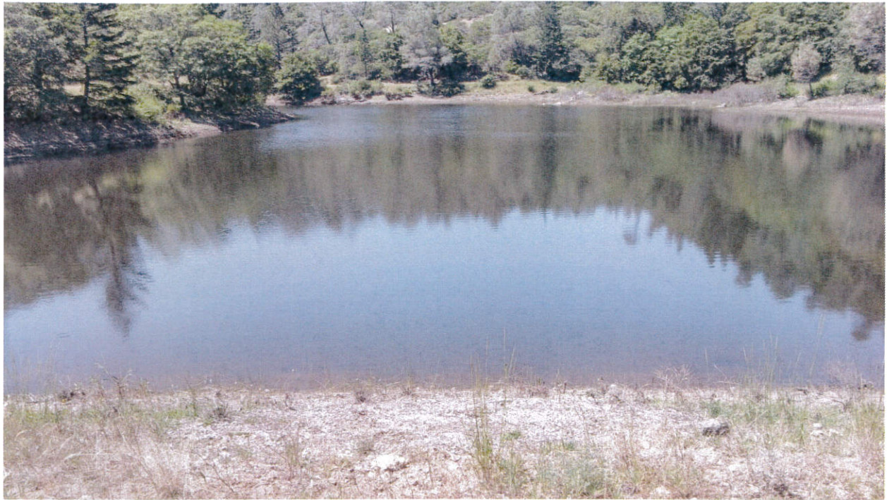
From Point of Rediversion at Cooksley Lake Dam (Map Point 8) Facing Upstream (May 22, 2017)
