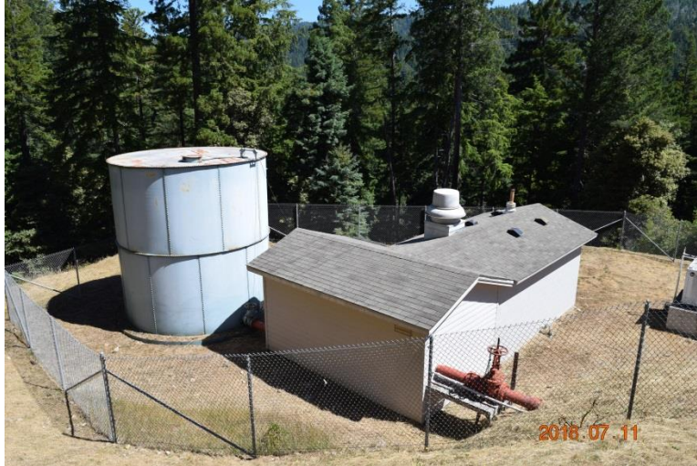
Booster Pump Station Dated July 11, 2018
