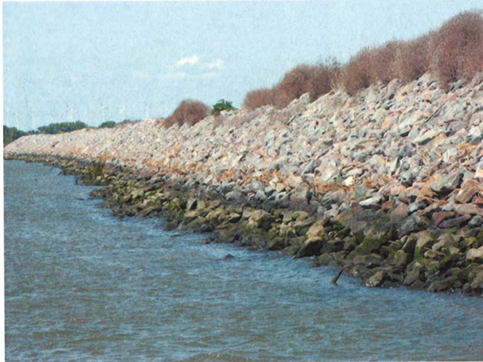
Figure 9. An example of the steep, rip-rapped banks of the lower San Joaquin River with limited or no vegetation.
