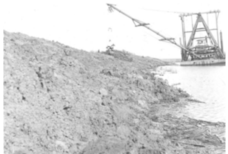
Construction of Yolo Bypass Levee
