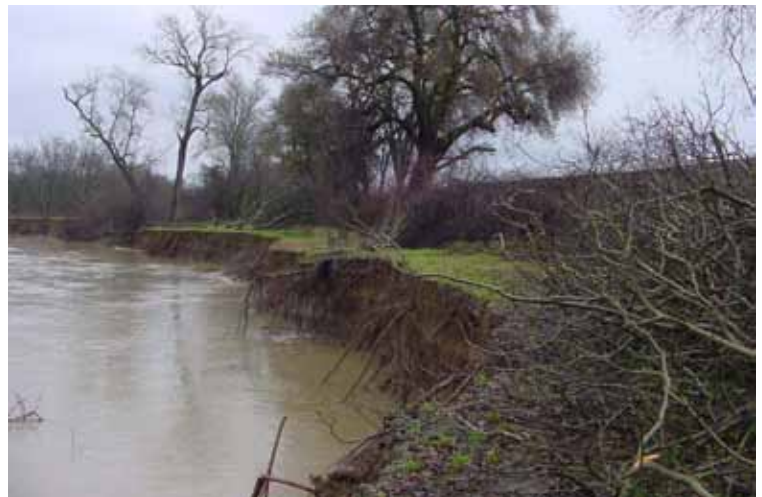
Erosion along the Sacramento River in January 2002
