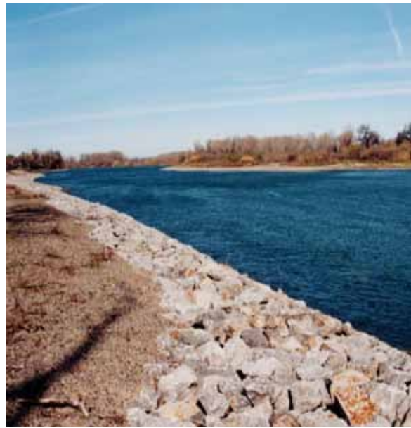
Typical Rock Revetment Along Sacramento River
