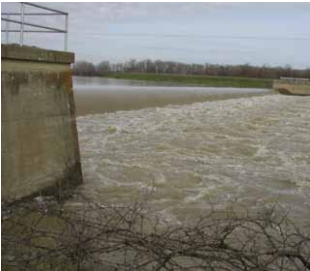
Floodflow over the Moulton Weir
