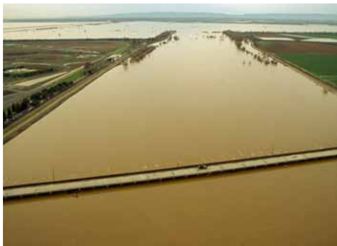
Water Flowing from Sacramento River to Yolo Bypass Through Sacramento Weir and Bypass
