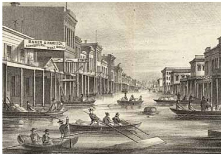
1862 Flooding in Sacramento
