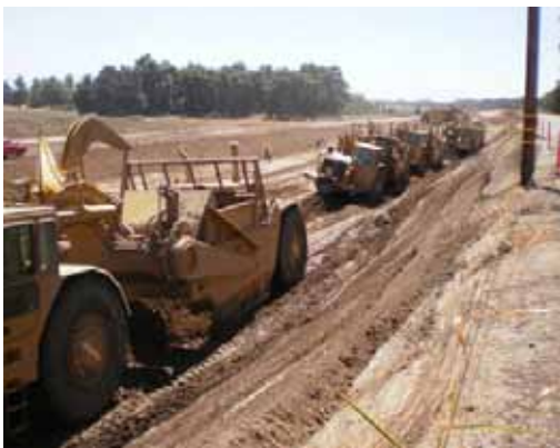
Levee Improvements in Natomas
