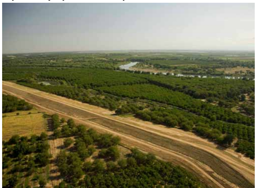
Feather River Setback Levee was Constructed for Multiple Benefits Including Improved Flow Conditions
