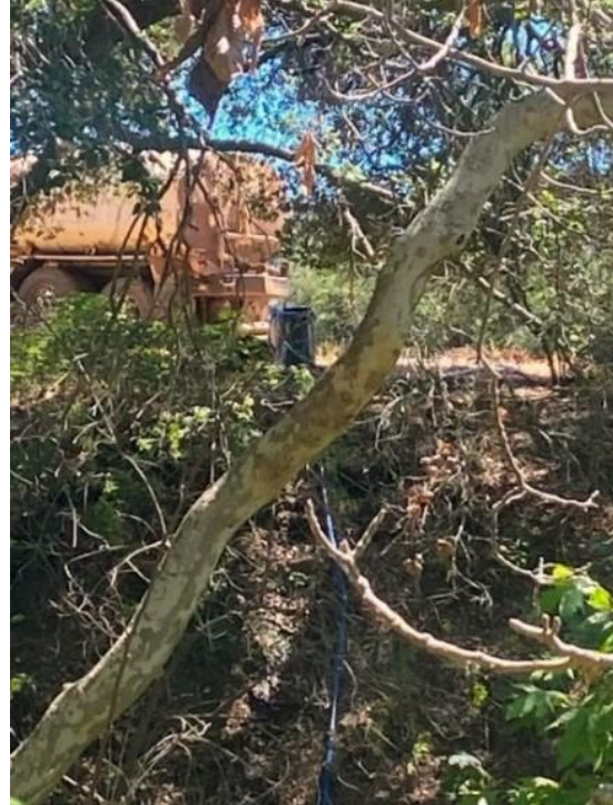
Figure 2 - Water truck carrying water from Calero Creek.
