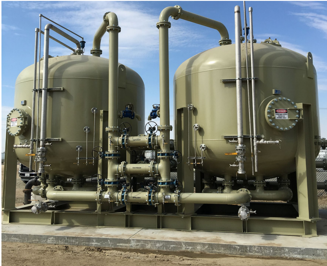
Figure 8. Example of Wellhead Treatment
