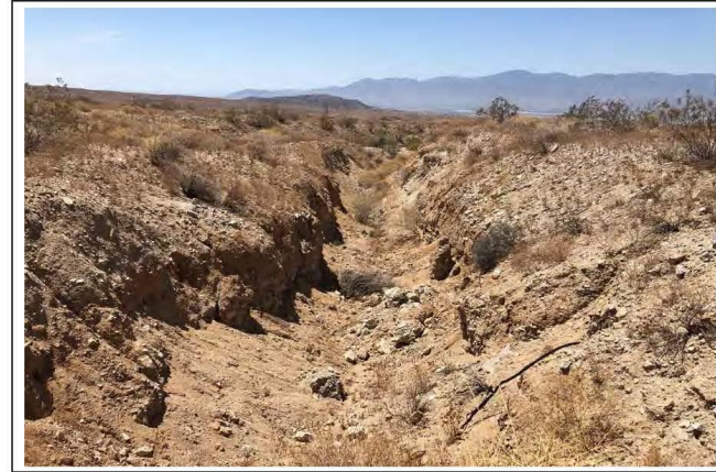
Photograph 18: View to the southwest of a non-jurisdictional erosional gully associated with an outfall structure at West Thermal Siphon [Work Area 11].
