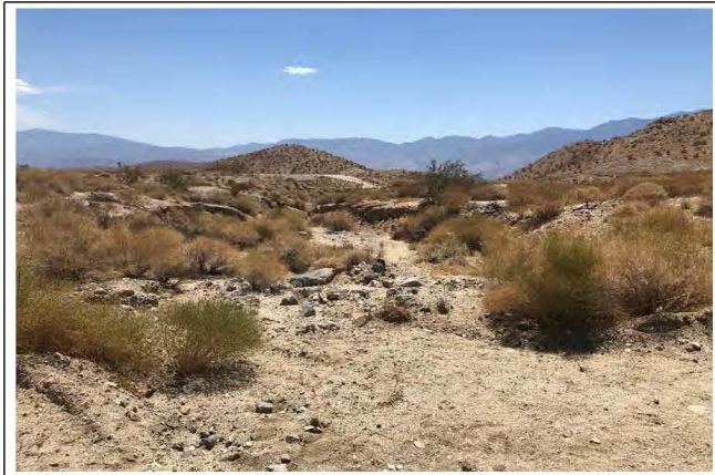
Photograph 19: View to the southwest of a non-jurisdictional erosional gully associated with an outfall structure at West Wide Canyon Siphon [Work Area 18].
