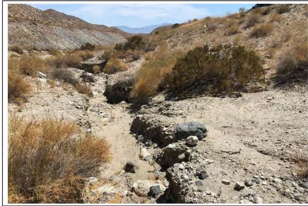
Photograph 5: View to the southeast (downstream) of Drainage F located at Long Canyon Siphon [Work Area 19].
