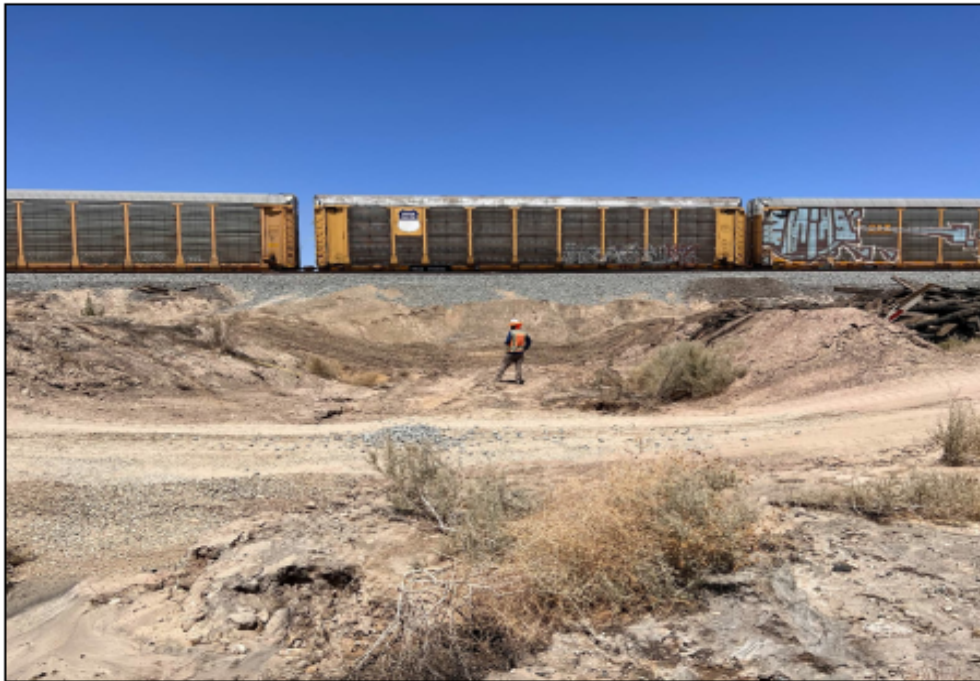
Photo 4. Southwest side of track facing fill repair location.
