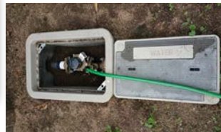
Smart Water Meter installed at Santa Teresa
