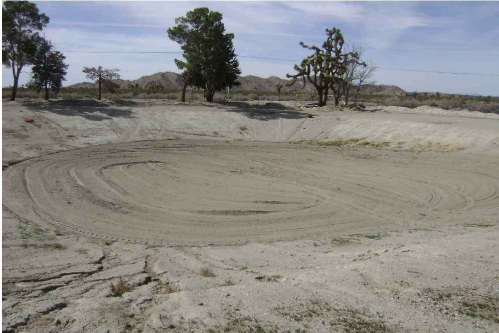
Photograph 10—Unlined pond for storm water runoff from corral area.
