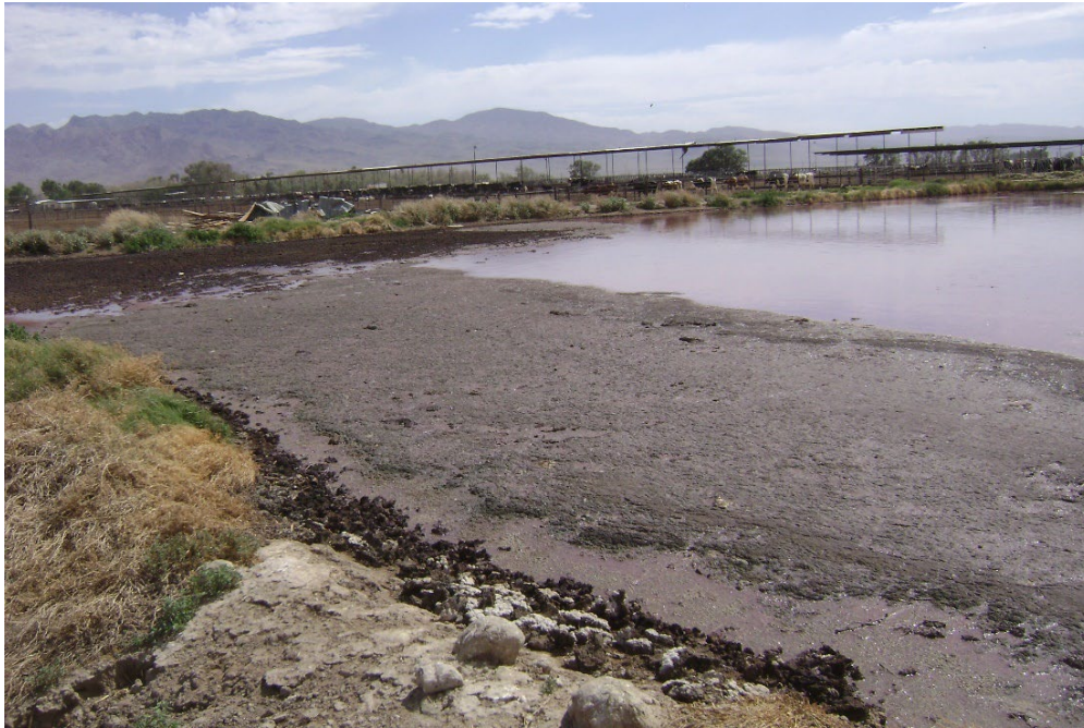
Photograph 9—Unlined disposal pond containing liquid and solid waste from dairy cow milk parlor wash water discharges.
