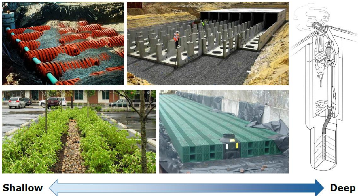
Figure 1 – Typical Stormwater Infiltration Systems
