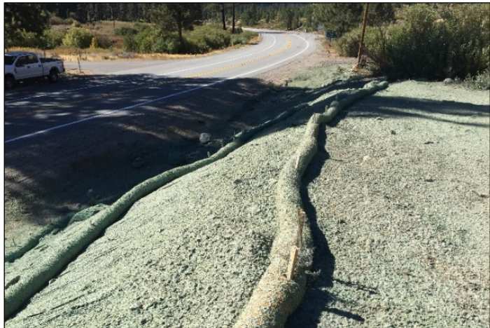
Erosion control measures installed following excavation (jute netting, straw wattles, and hydroseed), October 18, 2018.
