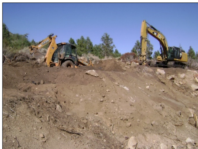
Second phase of soil excavation, September 26, 2018.
