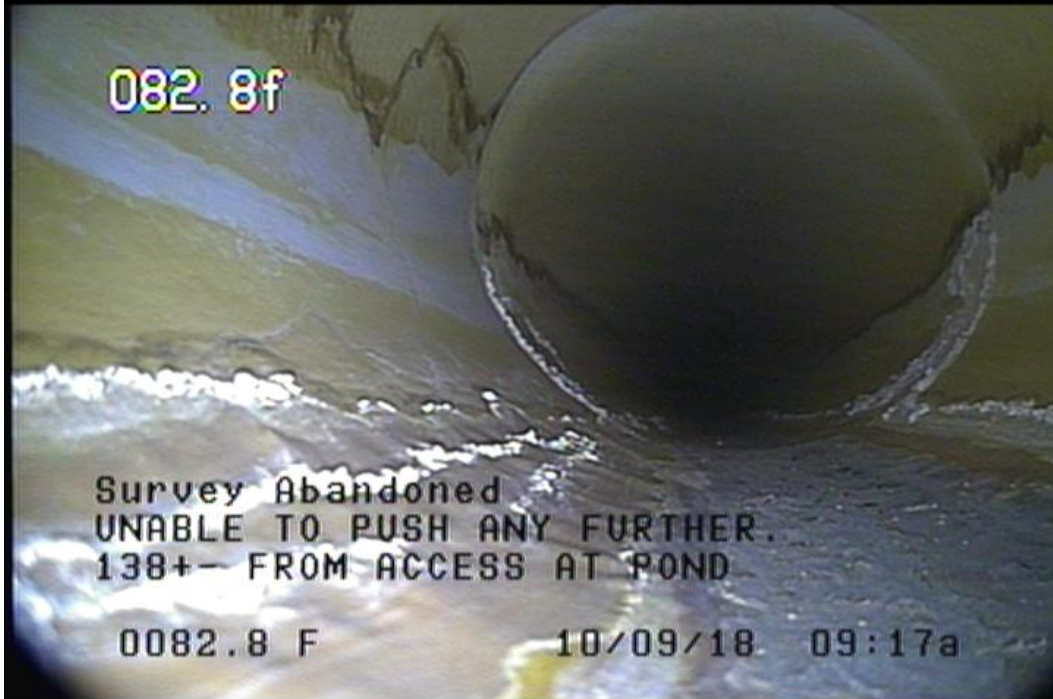
Photo 10 – October 9, 2018, Pond 3 overflow piping inspection
