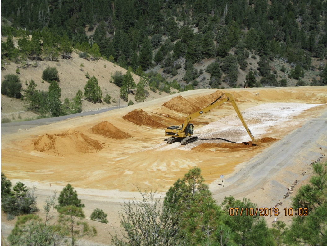
Photo 5 – July 10, 2018, sludge stockpile activities in Pond 3
