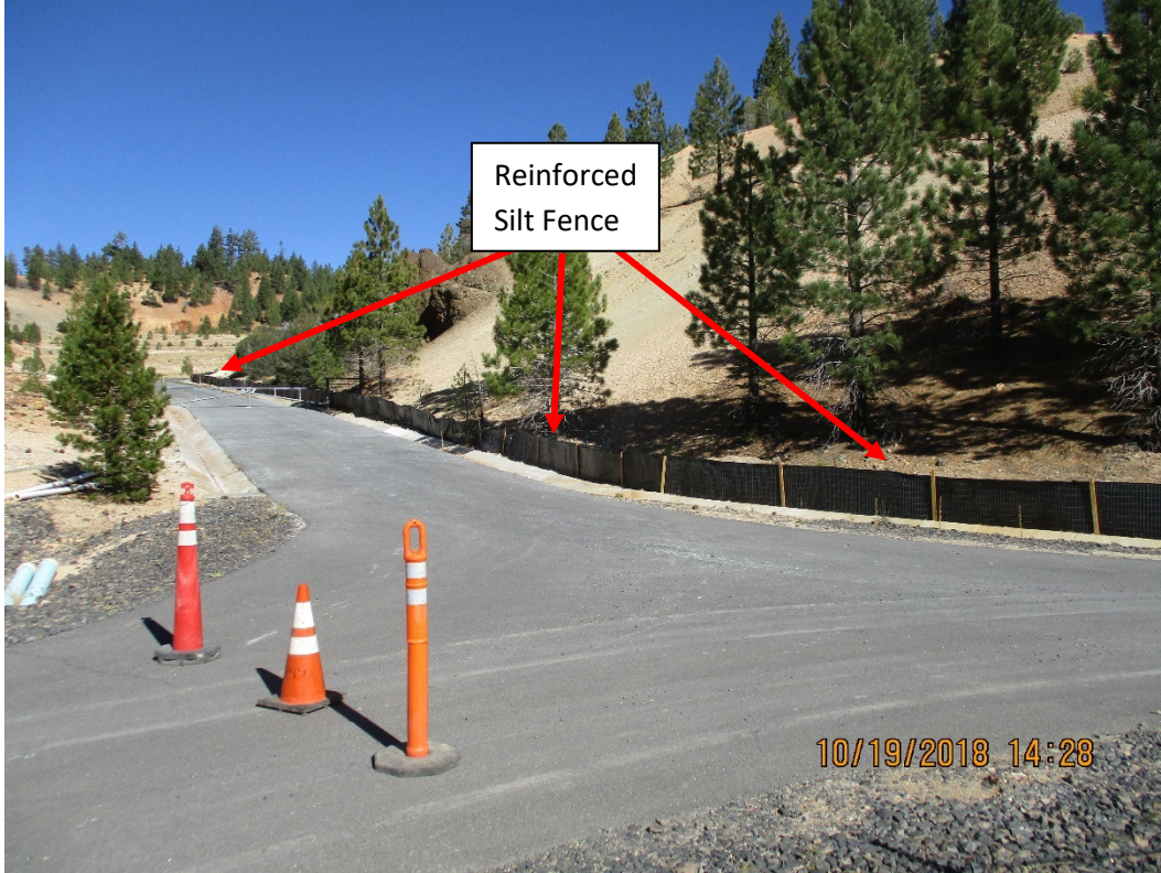
Photo 6 – October 19, 2018, Reinforced silt fence installed along the pit access road
