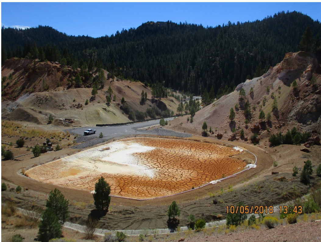
Photo 4 – October 5, 2018, Sludge generated during the 2018 treatment season is contained in the Pit Clarifier
