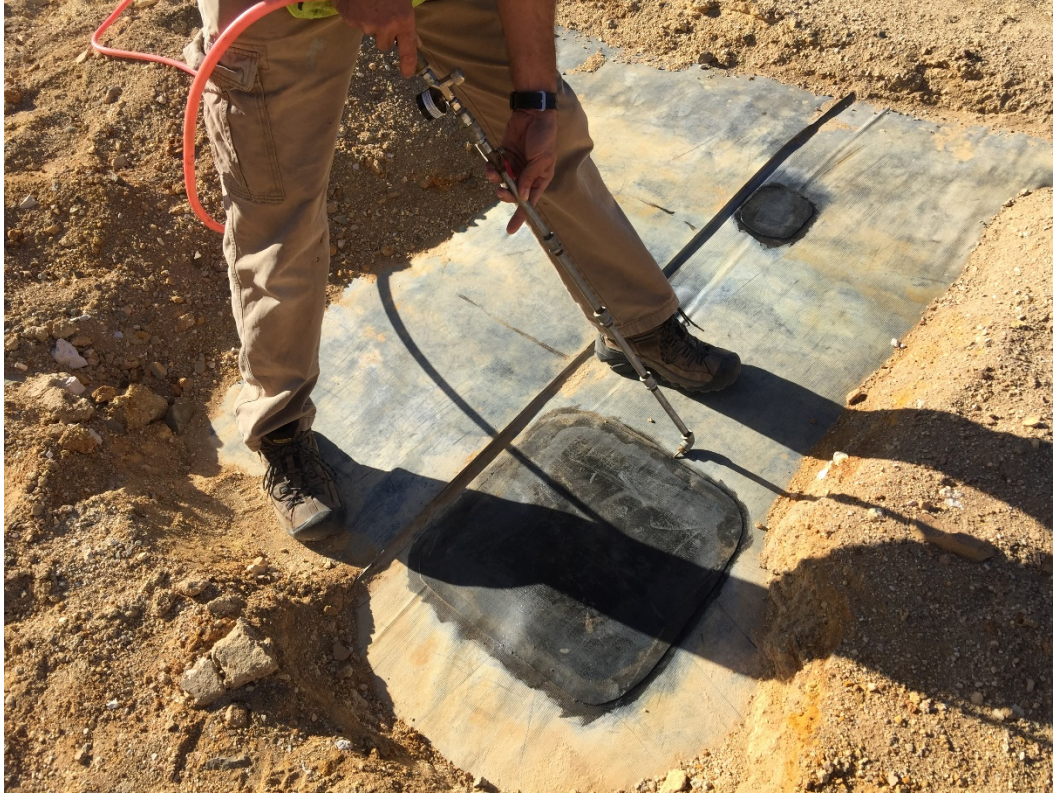
Photo 9 – October 10, 2018, Air lance testing of a Pond 3 liner patch
