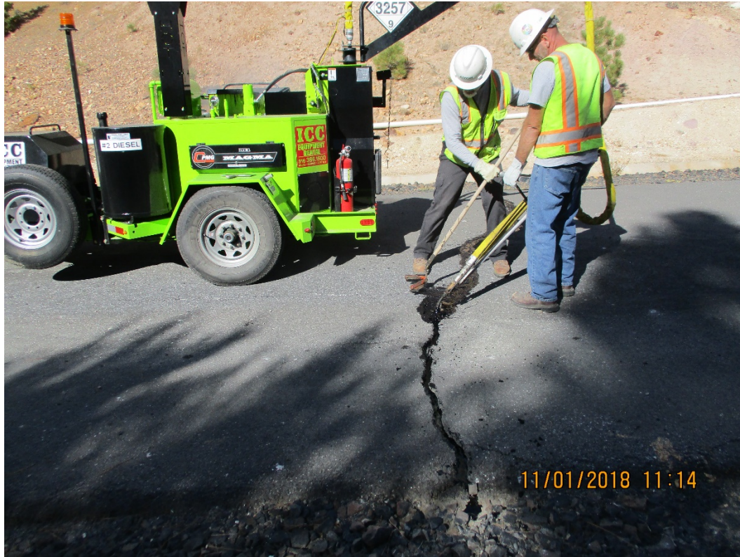
Photo 7 – November 1, 2018, Asphalt crack sealing on the pit access road
