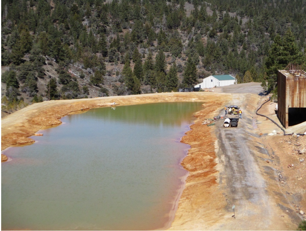
Photo 1 – April 20, 2018, Mobilization of RCTS and associated spring treatment equipment
