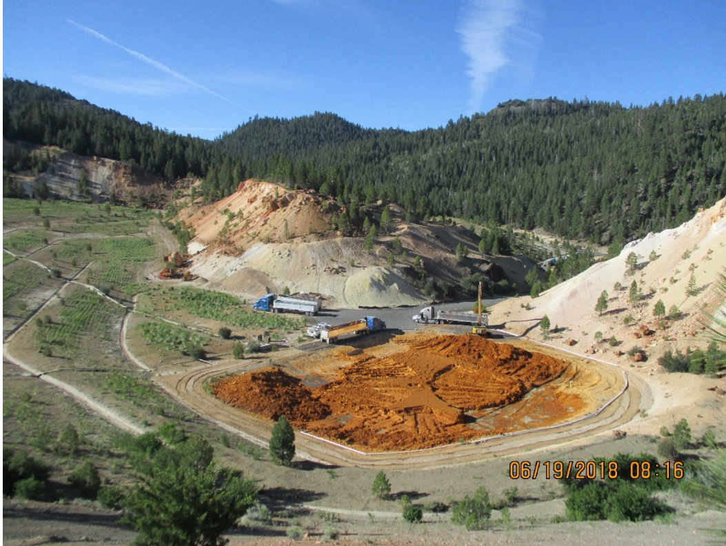
Photo 3 – June 19, 2018, Sludge stockpile and disposal activities at the pit clarifier
