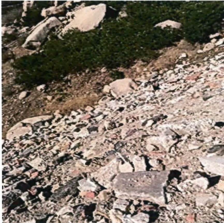
Figure 2: View facing down into the unnamed tributary of the construction debris stockpiling area.
