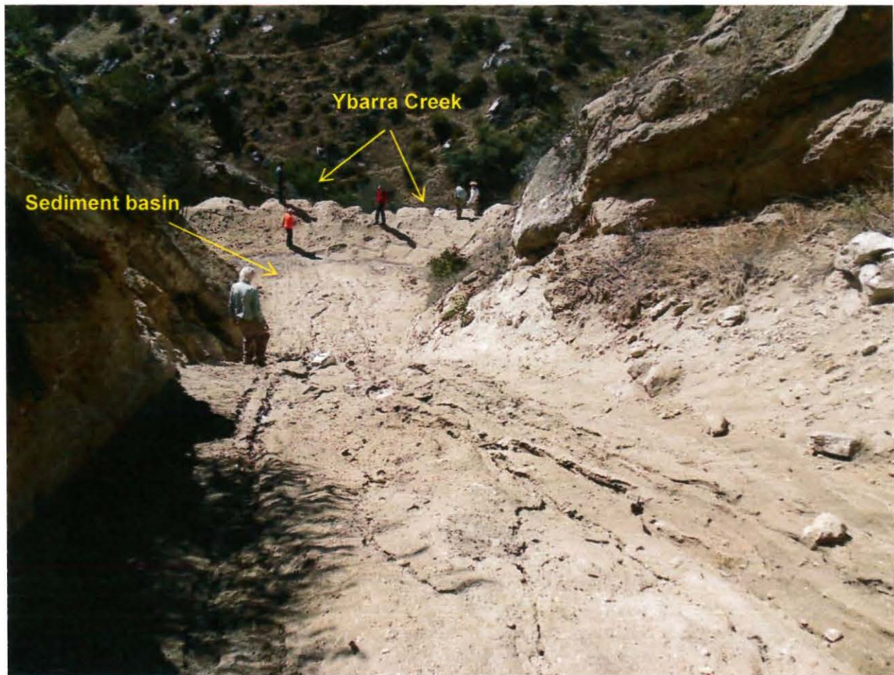
Photo 8. This photograph shows the toe of the slope at graded area 2 where a detention /desilting basin is located. The detention / desilting basin is built upon waste materials, some of which appears to be rebar-embedded concrete that spills into a trail that is within or immediately adjacent to Ybarra Creek.
