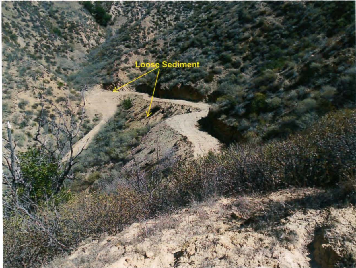
Photo 22. Road leading to Devils Creek with loose sediment and without BMPs.
