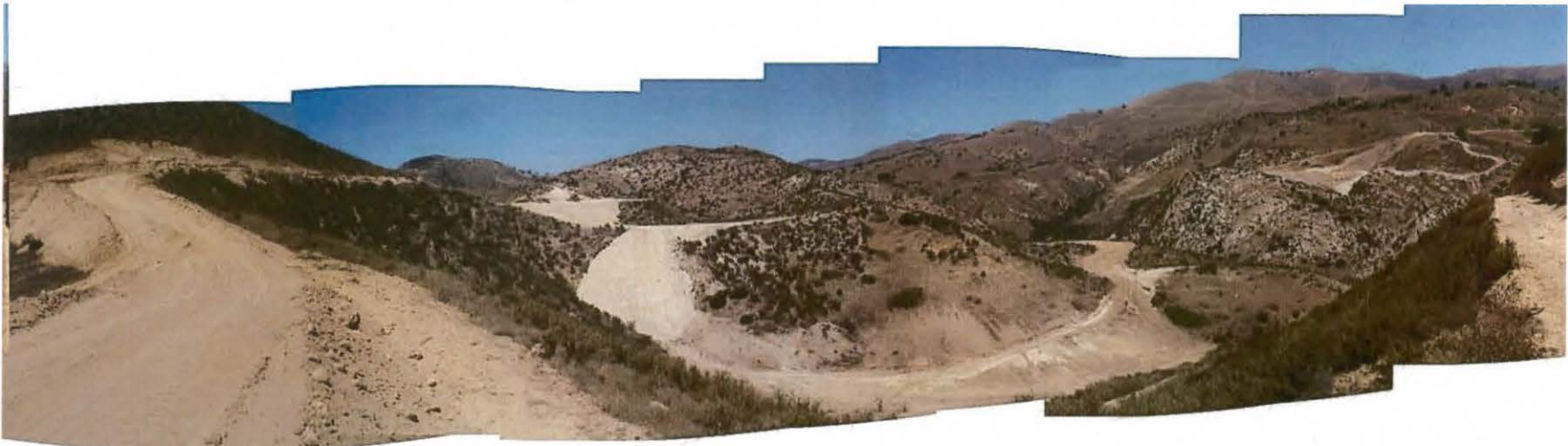
Figure 8. New area of activity for “concrete stockpiling.” On the left is the new road to the area and the “concrete stockpiling” area is in the distance. The steep slope ‘road’ in the center left leads to the ravine which Mr. Fishback says may be partly filled for a greenhouse. (Enrique Casas)
