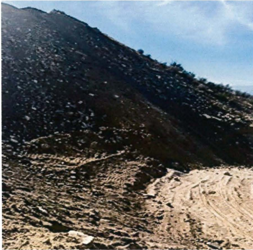
Figure 7. View of the east slope and construction debris stockpiling.
