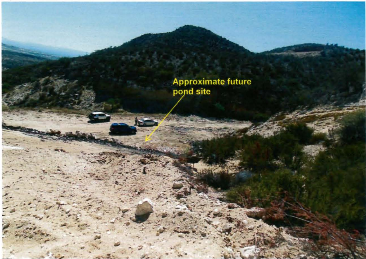
Photo 12. This photo shows graded area 3, and future site of a pond.
