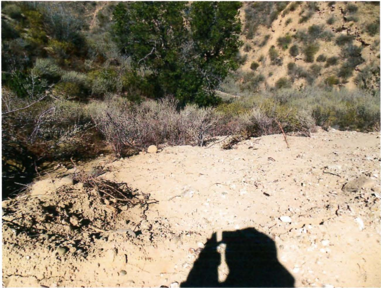
Photo 25. This is another photo of the road leading to Devils Creek with loose sediment and without BMPs.
