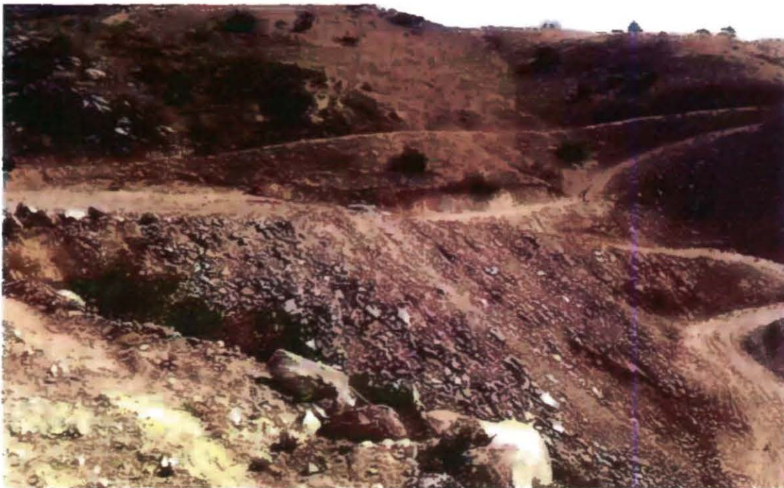
Figure 3: APN 2821-002-023. No significant changes were observed in this area, comparing to what was observed during the inspection on May 4, 2015.
