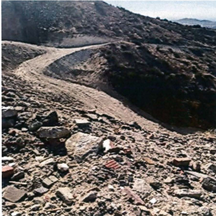
Figure 1: View facing east, of the stockpiling area within the unnamed tributary in Brown's Canyon.
