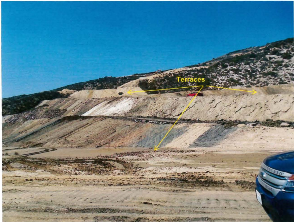
Photo 31. This photo show graded area 1 and added terraces.
