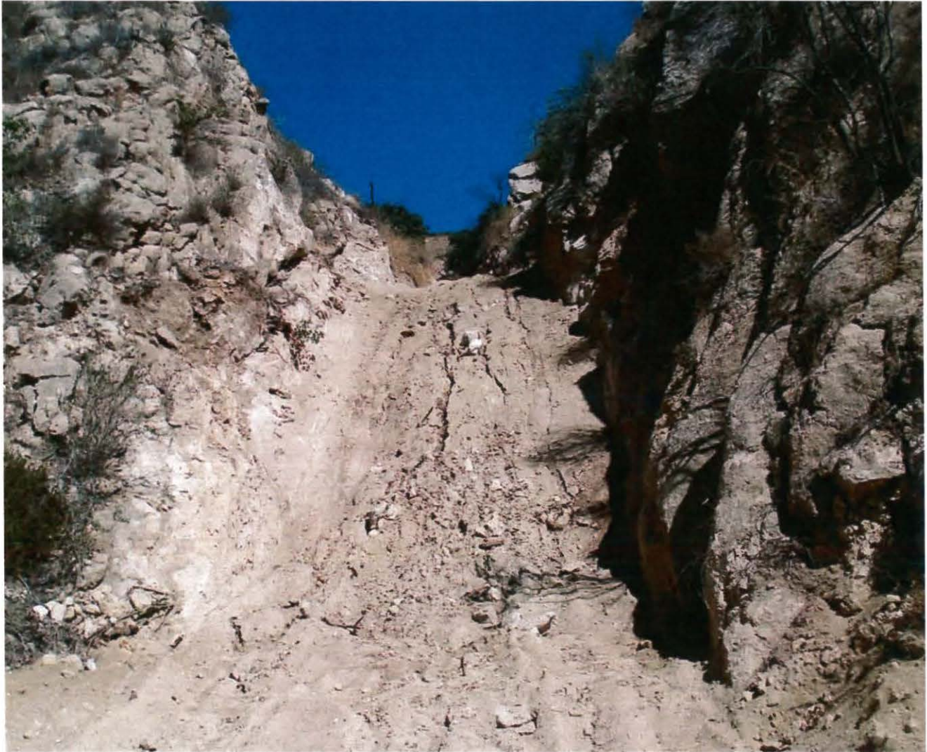
Photo 9. The graded area 2 is so steep that it cannot be freely walked down in places. The steepness and angle of repose entrains some of the material that falls from above, and contained within the steep walls of the ravine.
