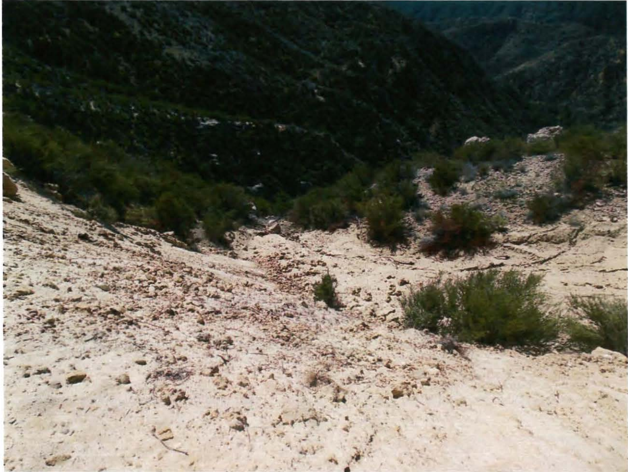
Photo 19. This photograph shows the down gradient of photo 13, above. This area has loose sediment without best management practices (BMPs), and poses a potential for loose sediments to dislodge into the canyon below.
