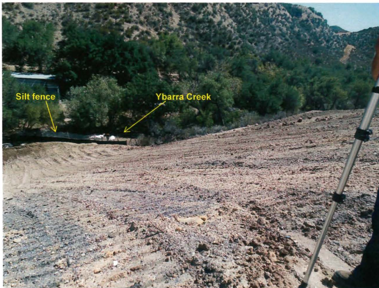
Photo 34. This photo shows another view of Ybarra Creek and the slope from photo 28, above, and a silt fence that was being installed at the time of the inspection.
