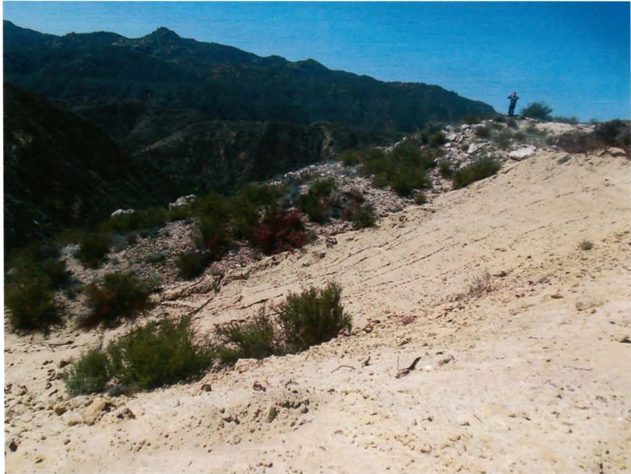
Photo 18. This photograph shows a graded area where vegetation was removed.
