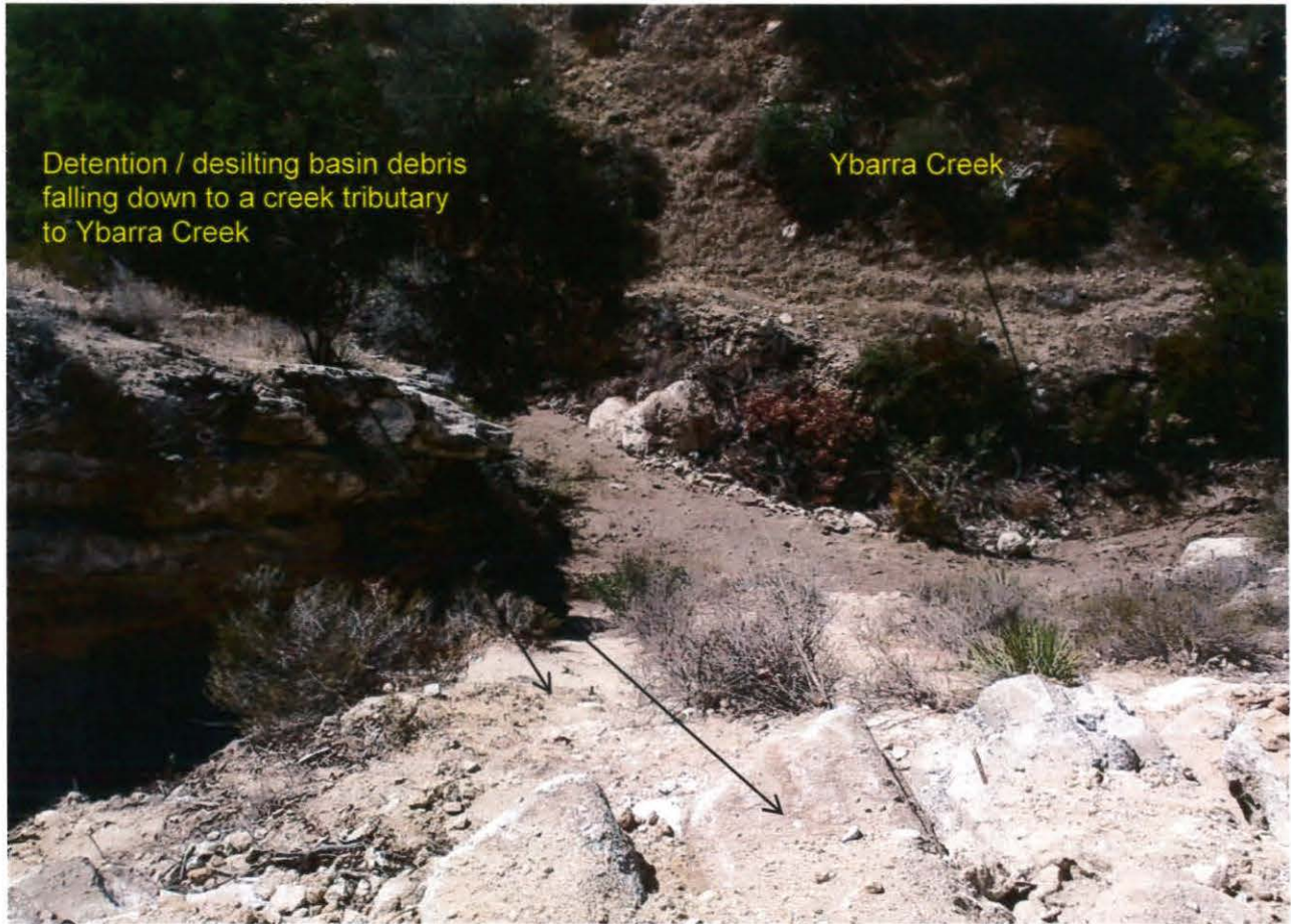
Photo 11. The detention / desilting basin is built upon waste materials that spill into a trail that is within or immediately adjacent to Ybarra Creek.
