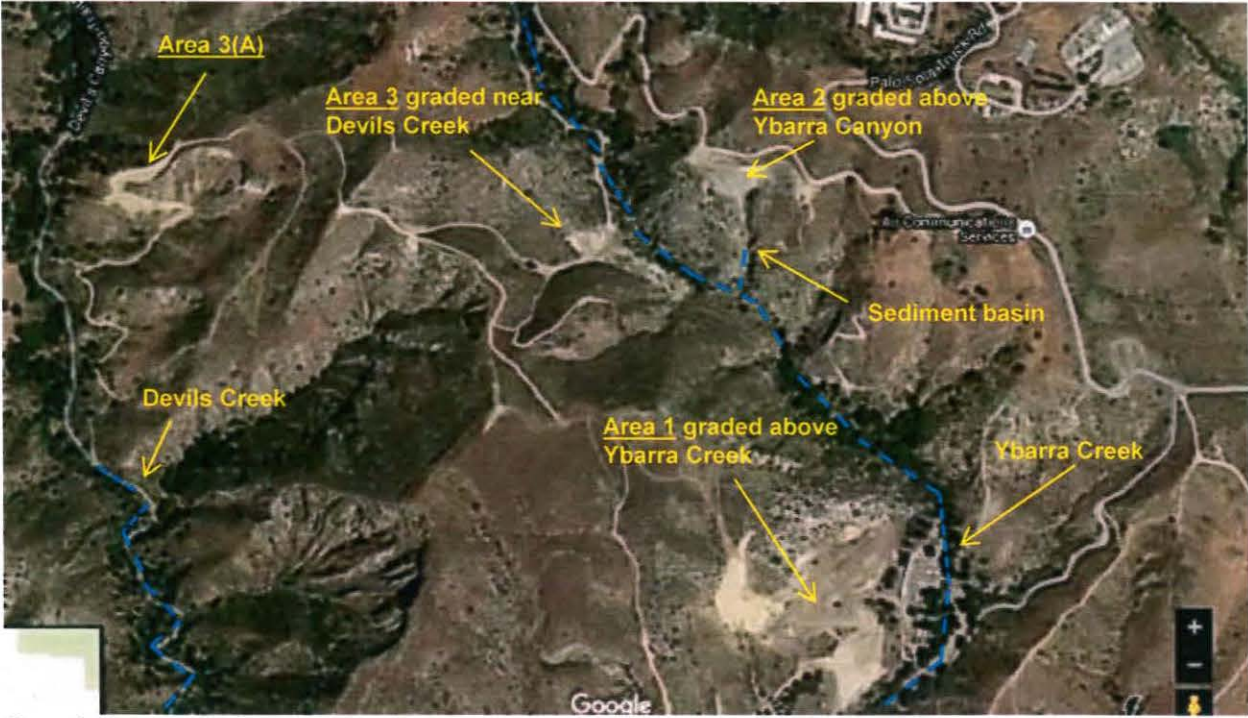
Google Image 1. Image showing areas that have been graded at the Site.
