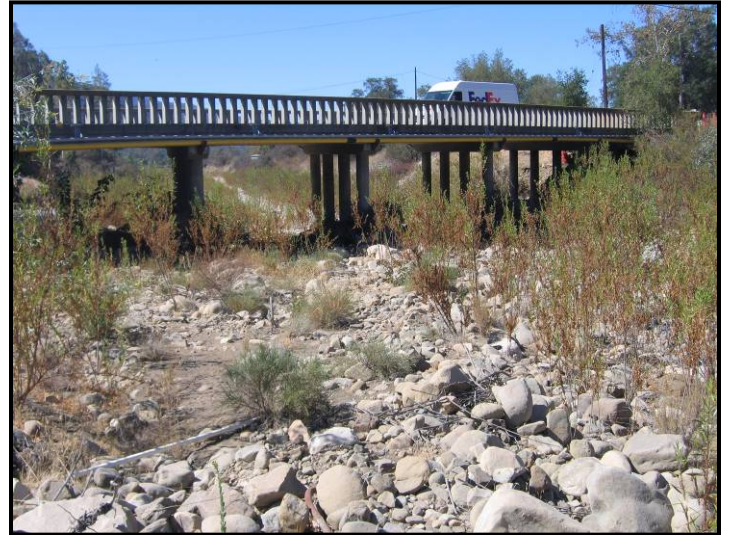
View downstream at the Grand Ave. bridge
