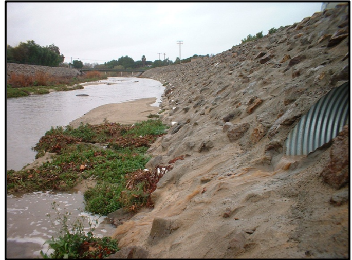
View of pipe discharging into Arroyo Simi
