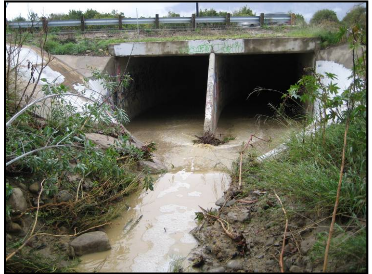
View of site (S) toward Hwy 126 bridge
