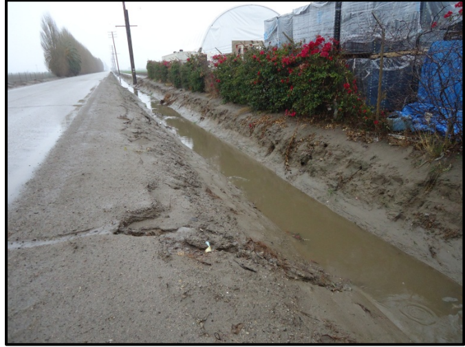
View at site looking upstream
