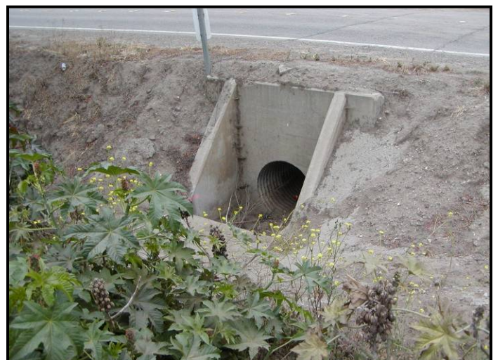
View toward SE of culvert draining runoff from CSUCI campus.
