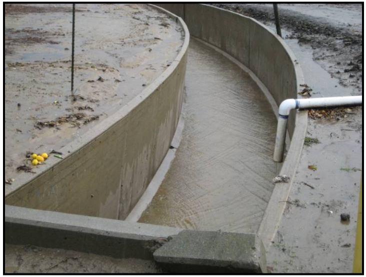
View upstream (NE) from sampling location
