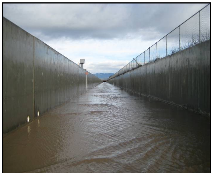
View upstream (NW) facing gage #781
