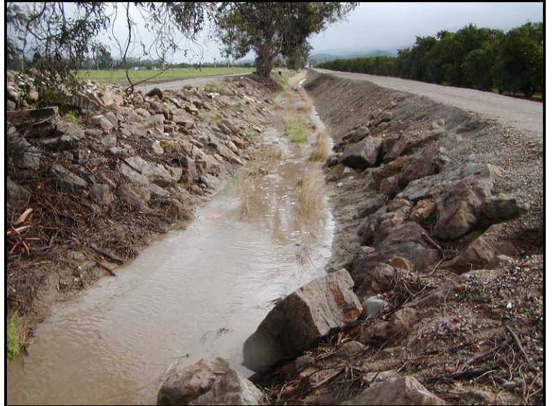
View of site looking upstream
