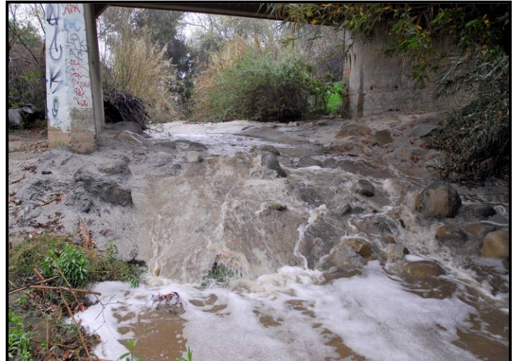
View upstream at the bridge pier
