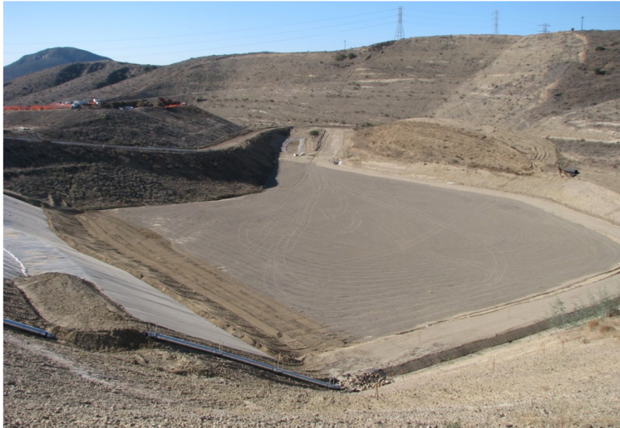
New Stage III-B Unit at the Sycamore Landfill
