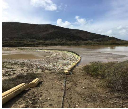
Trash captured in Goat Canyon sediment basins trash interceptor device.
