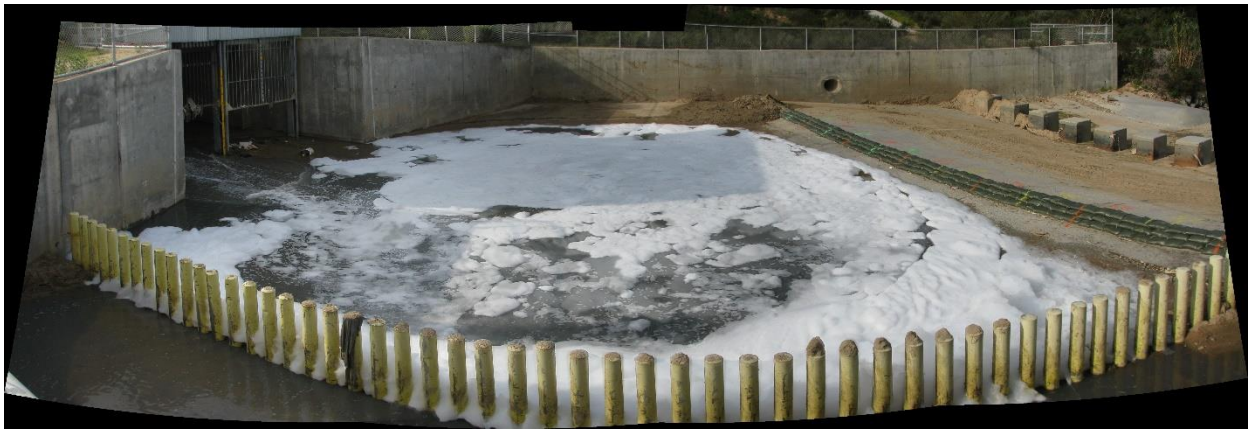
Figure 5: Smugglers Gulch Diversion Structure on January 16, 2020, Photo by San Diego Water Board
