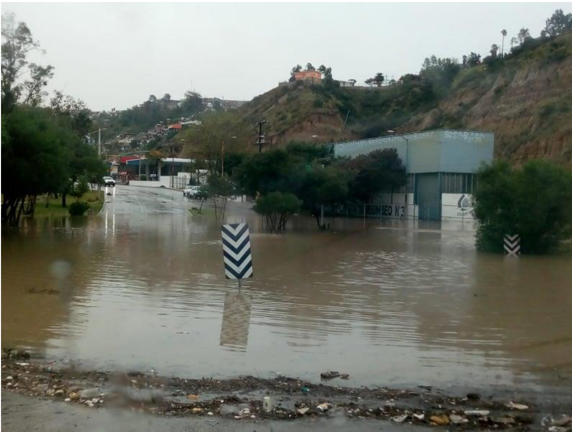
Figure 3: CESPT Pump Station No. 3 in Matador Canyon, Tijuana Mexico, Ground View, Photo provided by IBWC on December 26, 2020
