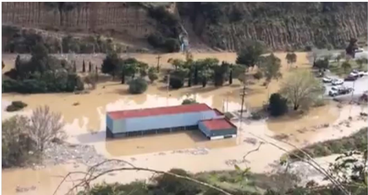
Figure 4: CESPT Pump Station No. 3 in Matador Canyon, Tijuana Mexico, Top View, Photo provided by IBWC on December 26, 2020
