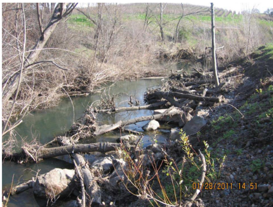
Figure 2. As part of the restoration of the Rutherford Reach on the Napa River, large woody debris was successfully placed in the river to enhance in-stream habitat.
