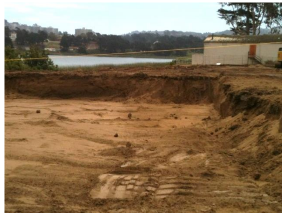
Figure 2b. Pacific Rod and Gun Club site during cleanup.
