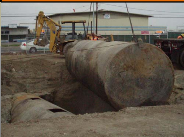
Photo 1: Excavation of 10,000-gallon gasoline UST
