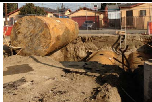
Photo 2: Removal of three 10,000-gallon USTs
