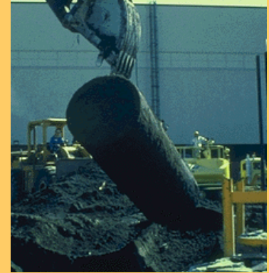
Photo 2: UST being removed
