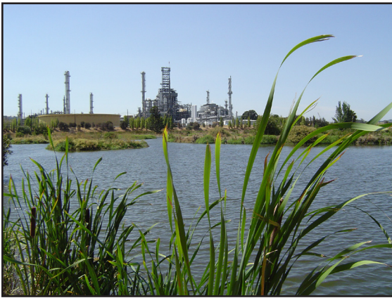
Mountain View Sanitation District Flushing Pond (Treated Wastewater) (Photo courtesy of State Water Resources Control Board)
