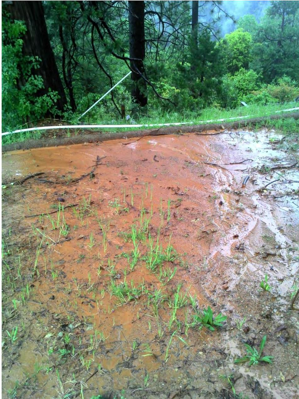
Photo 4. Main Access Road exhibiting heavy sheet flow, erosional scarring, and lack of erosion control measures.
