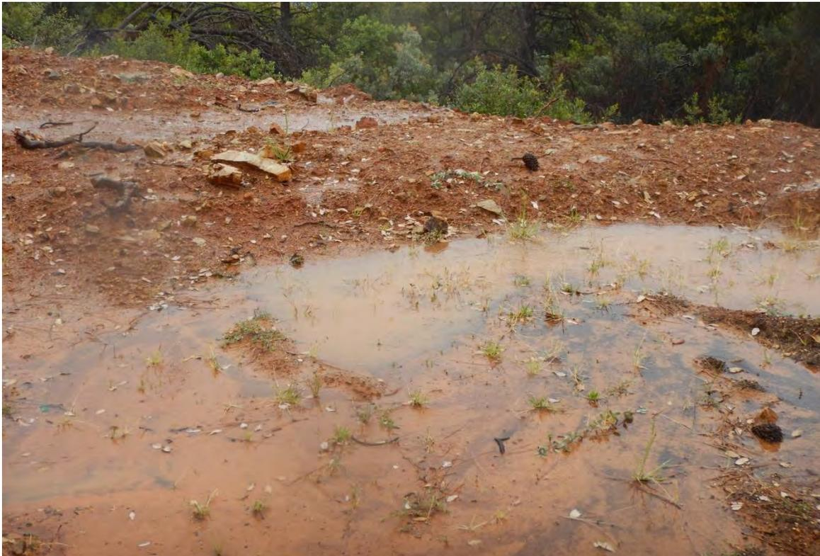
Photo 59: Unprotected cut-slope from second terrace to third terrace.
