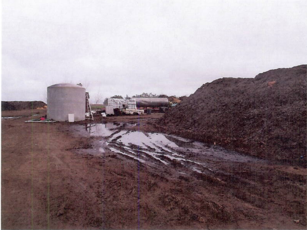
3/3/2016 – Compost pile with standing water.
