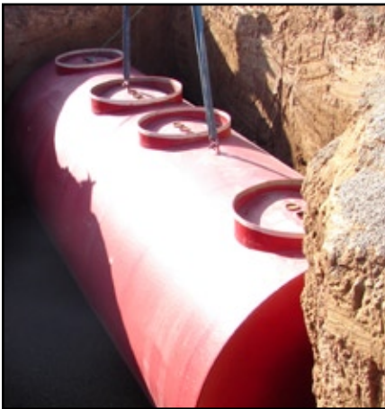
Water Boards Photo Underground storage tank
