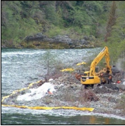
Photo by Earl Ambrosini, Beacom Construction Co. Used with Permission/ Region 1 Crews clean up along the Smith River after 4,000 gallons of fuel spilled.
