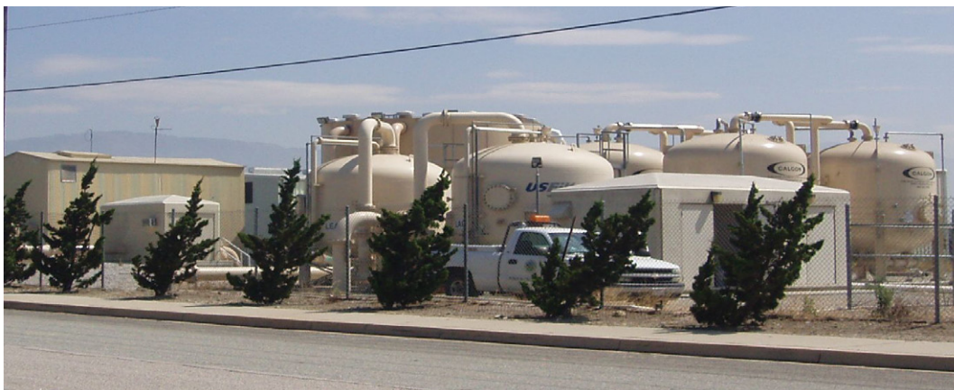
The perchlorate and TCE treatment system installed by the County of San Bernardino at the City of Rialto's Well No. 3. Photo by: Kamron Sarem, Regional Water Board staff.
