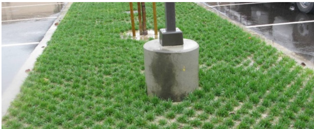
Low impact development in a Ventura County parking lot, using landscaping to capture and treat stormwater runoff (known as bioretention).
