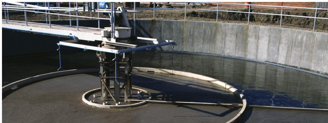
Wastewater treatment plant clarifier, which separates solids from partially treated wastewater. Stock Photo.
