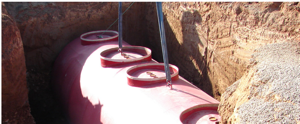
Underground storage tank. Photo by: Regional Water Board staff.
