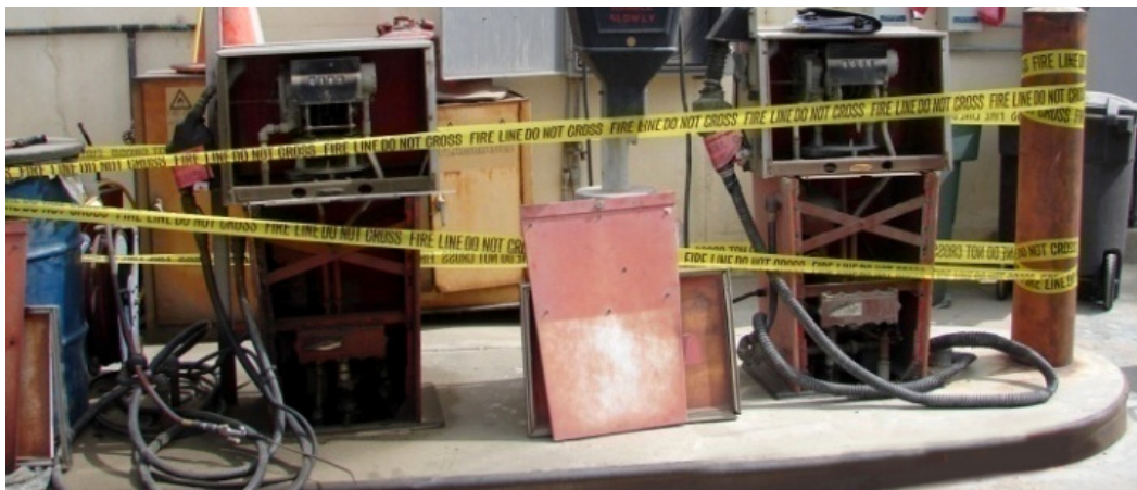
Fueling station for Long Beach City vehicles with two closed fueling dispensers, located next to the beach, with no required containment.
