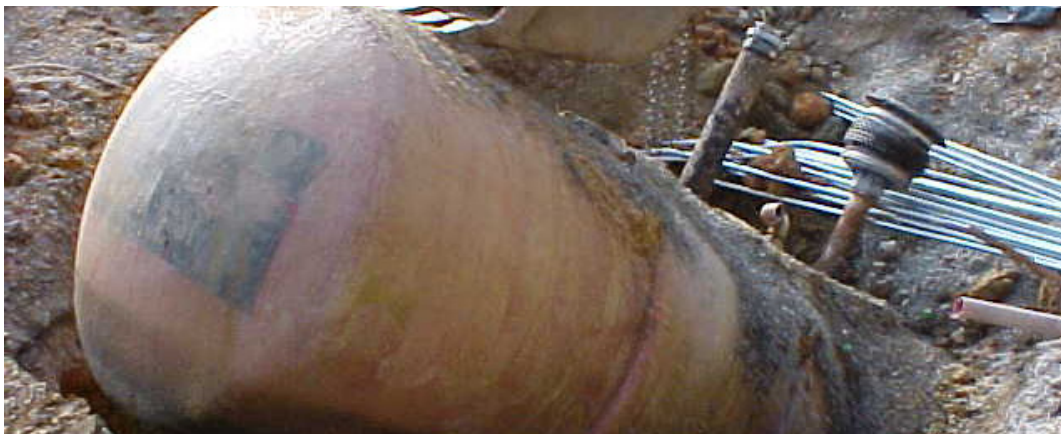
Removal of a leaking underground storage tank from an excavation. Stock Photo.
