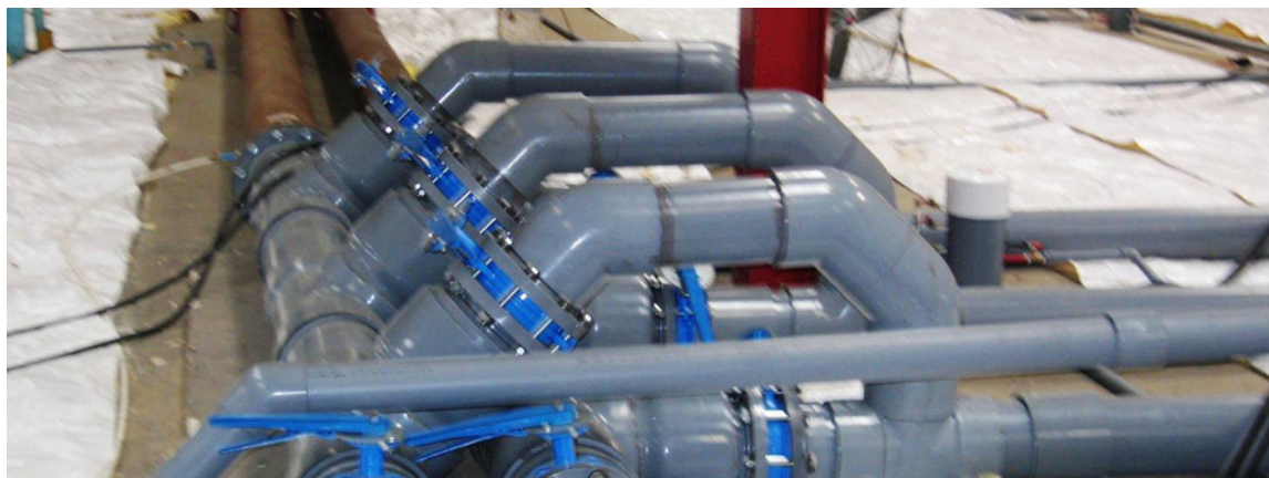
Air flow lines and insulation being installed to treat contaminated soil and shallow groundwater at the former Gillette/PaperMate facility in the City of Santa Monica.
