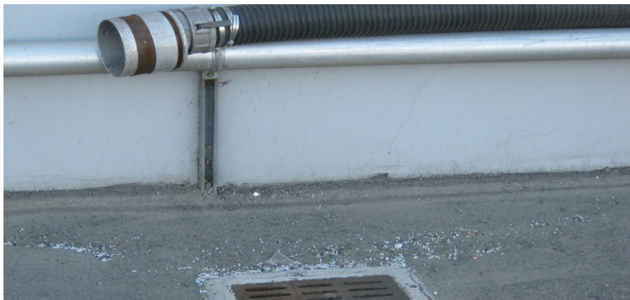
Pre-production plastics are transferred during delivery using this hose situated directly above a storm drain inlet in the City of Corona, Riverside County.
