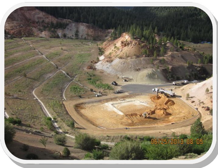
Leviathan Mine Sludge Clean Out, Lahontan Regional Water Board
