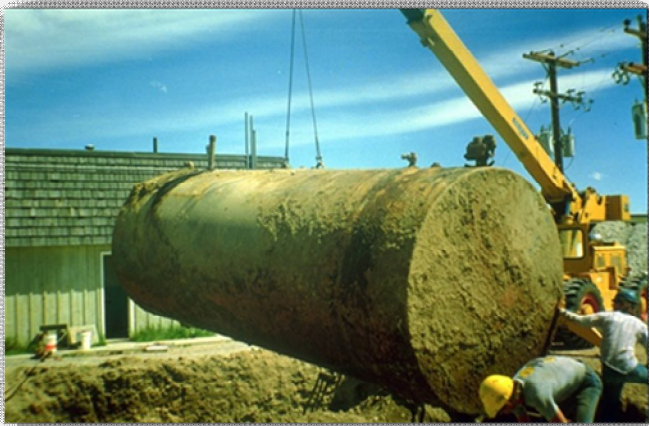
Underground Storage Tank Removal, Water Boards
