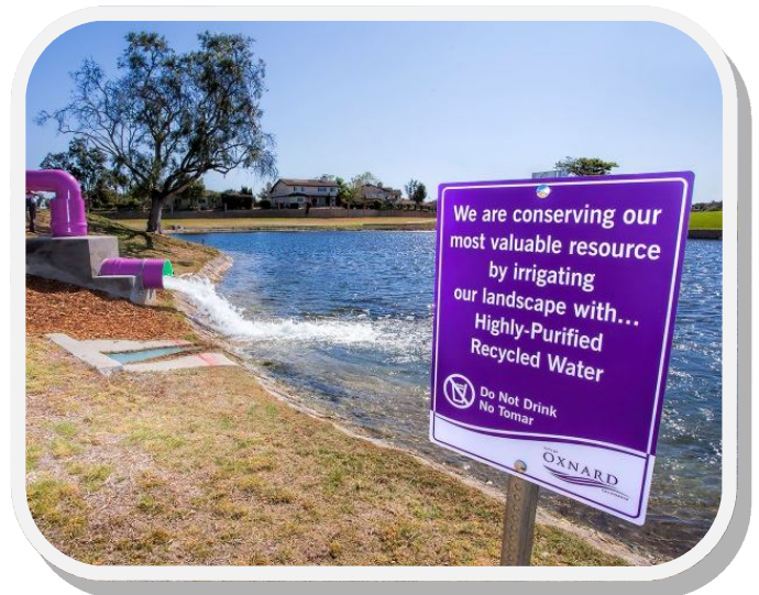
City of Oxnard Recycled Water Irrigation Impoundment, WaterReuse
