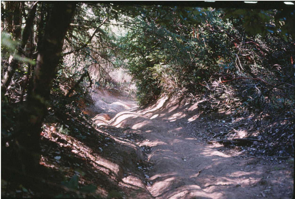
Figure 5.4 Abandoned throughcut logging road with deep rilling in the El Corte de Madera Creek Preserve (photo taken in 1994)
