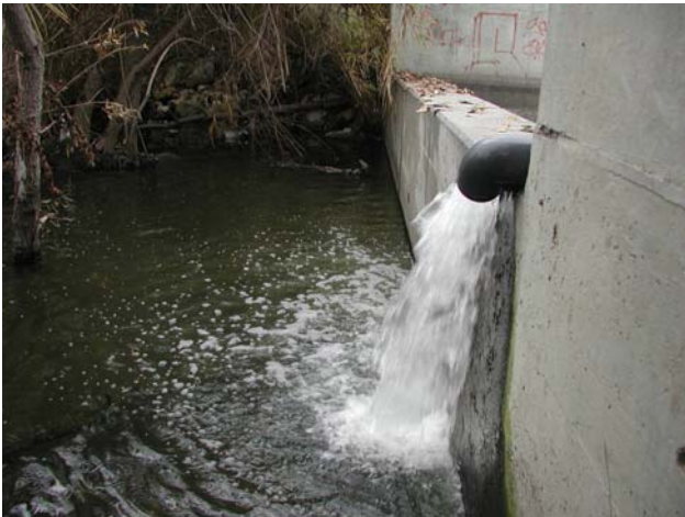
Figure 6.A Energy Dissipater End Wall and Discharge Point for Treatment System Effluent
