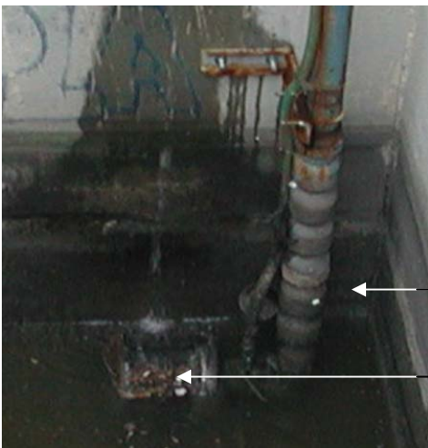
Figure 6.A Energy Dissipater End Wall and Discharge Point for Treatment System Effluent
