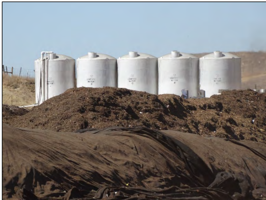
Water Tanks, Piles of Composted Materials, Covered Piles
