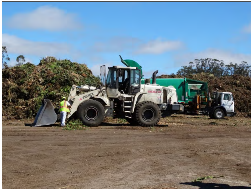
Feedstock Piles, Earthmoving Equipment
