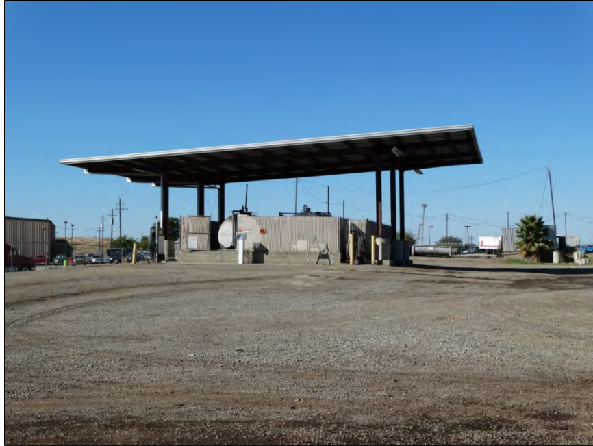
Co-Located at a Transfer Station which Manages its Own Fleet: Fueling Structure, Outbuildings, Area Lighting
