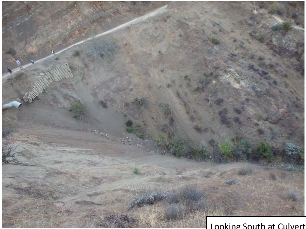
Looking South at Culvert
