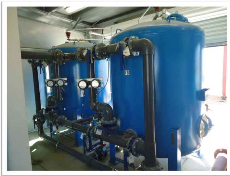
Part of the new water system at Aerial Acres.
