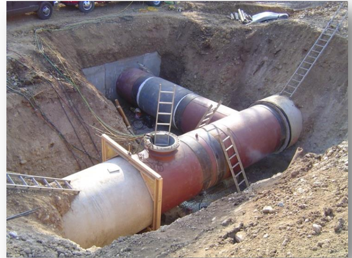
Pipelines 3 and 4 Interconnect
