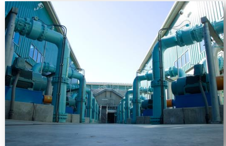
Twin Oaks Valley Water Treatment Plant
