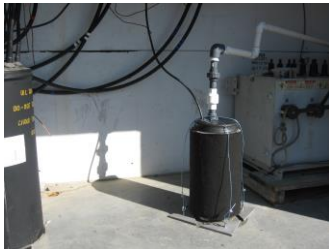
Installed ECO Pump
