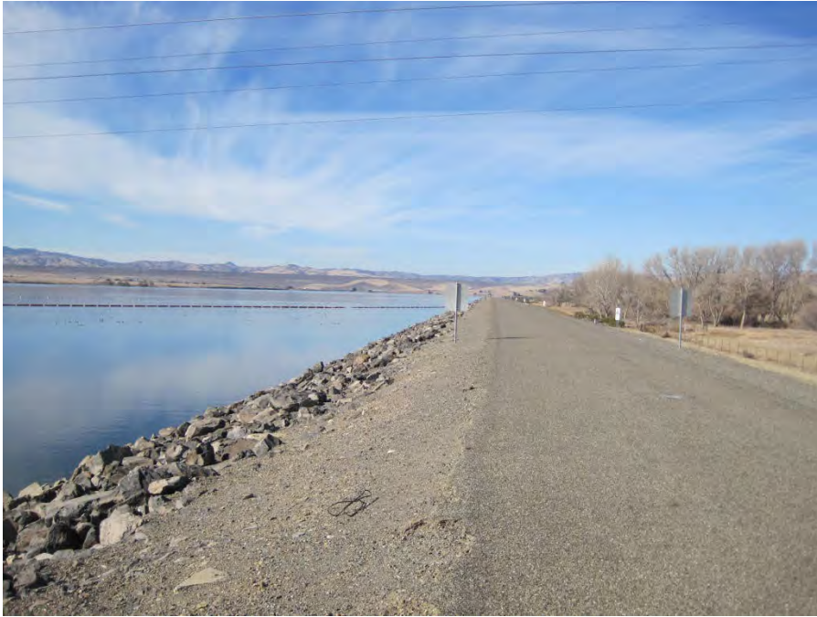
Photo 1. Facing north. Photo depicts the eastern shoreline of the forebay lined with crushed rock, greatly limiting the potential for vegetation or suitable plant and wildlife habitat to establish.
