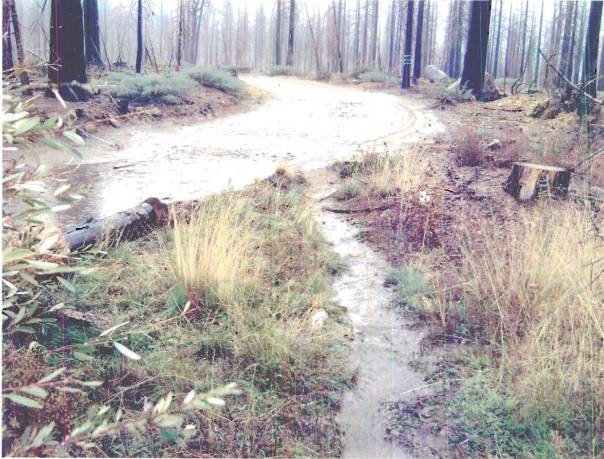
**Photo 5: Sediment-laden stormwater discharging from road and crossing 11 into Angora Creek. No erosion control structures are installed.**
