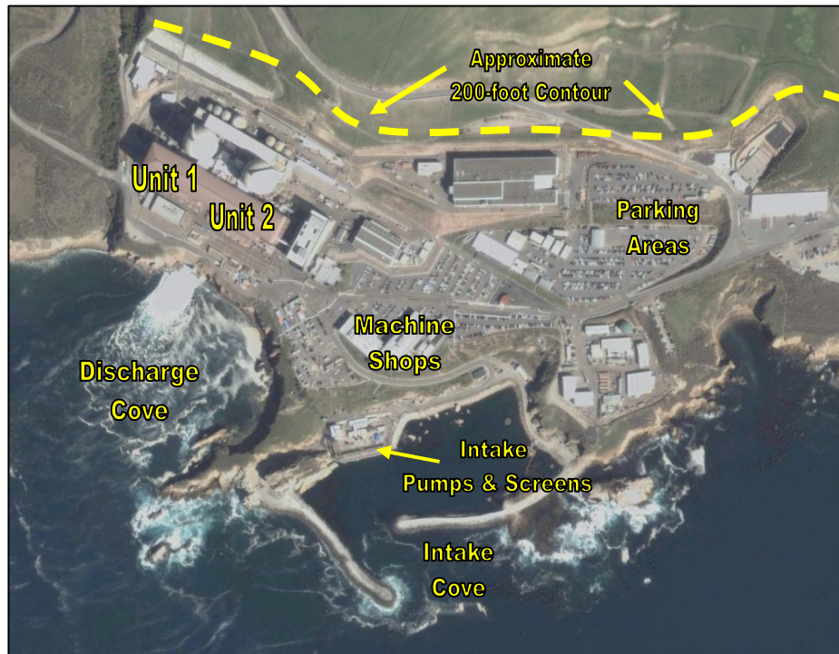
Figure C-3. Lower Site Overview
