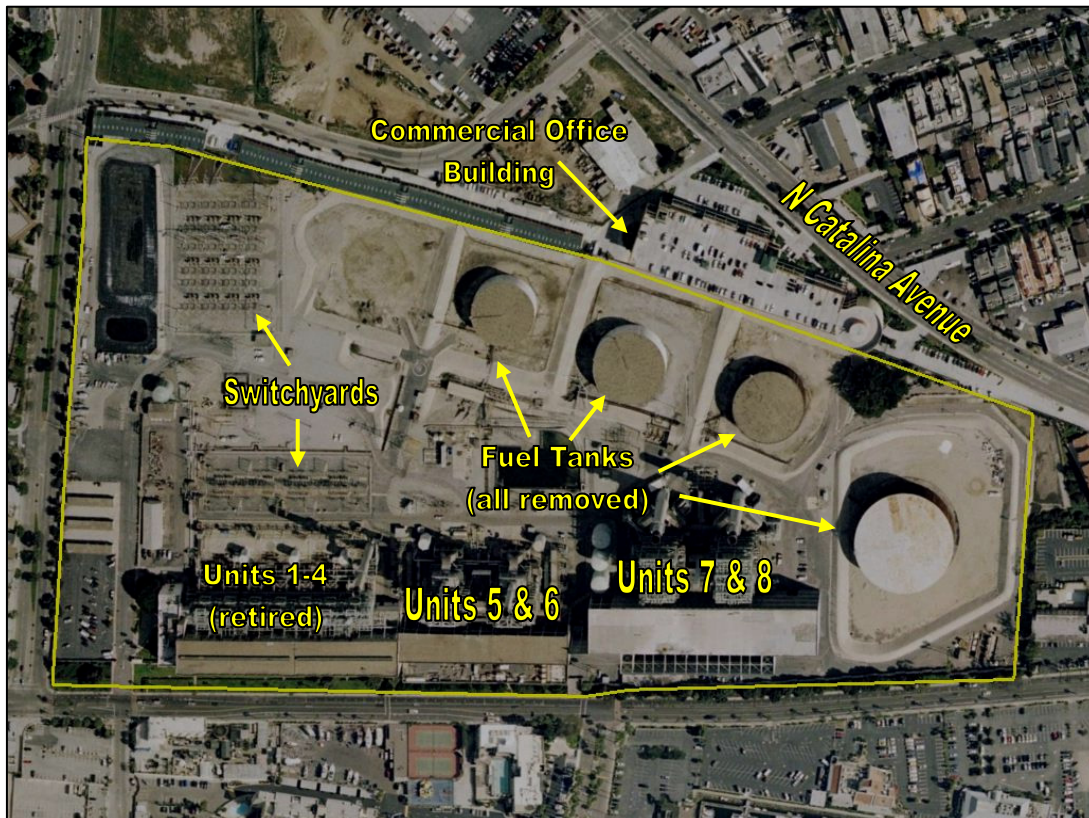
Figure M-2. Site View
