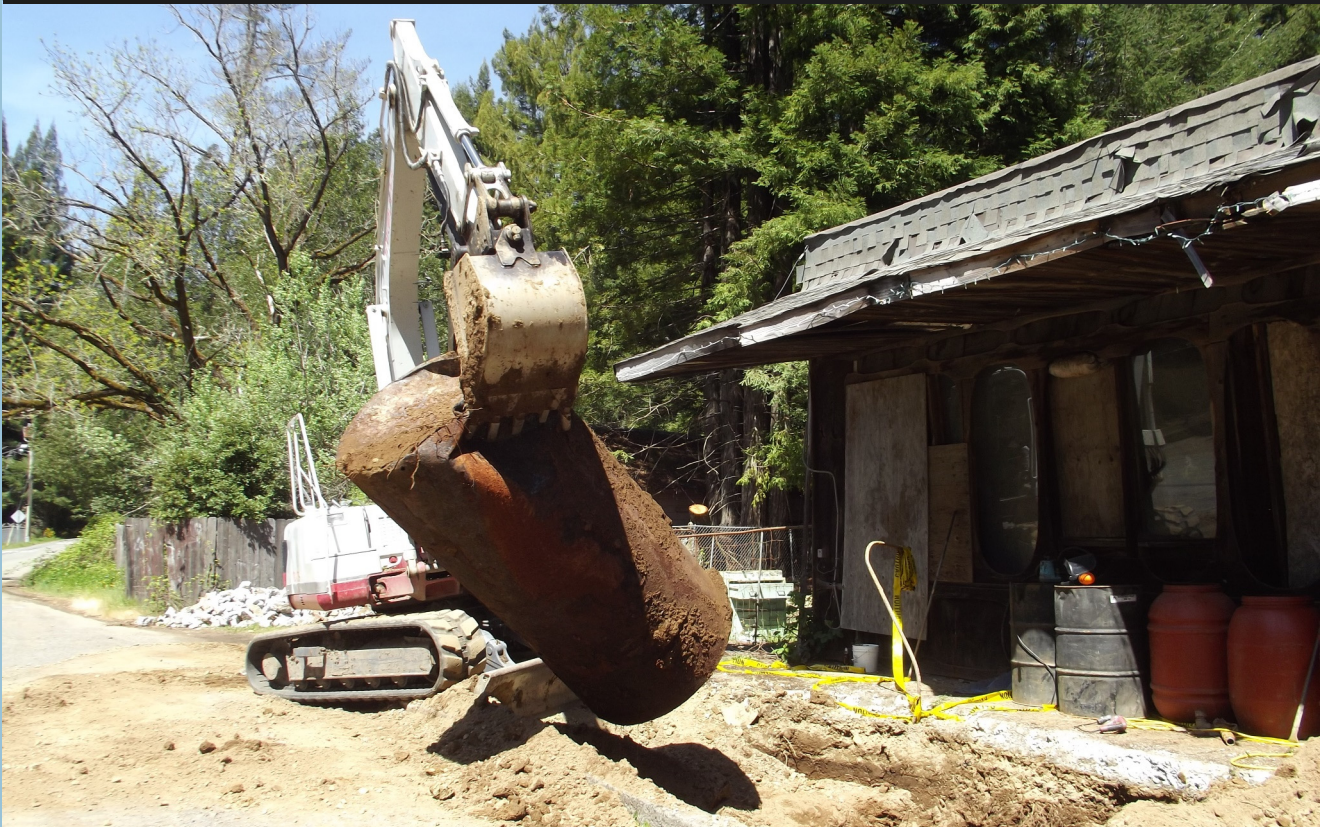
Photograph 1: UST being removed by a track-mounted excavator
