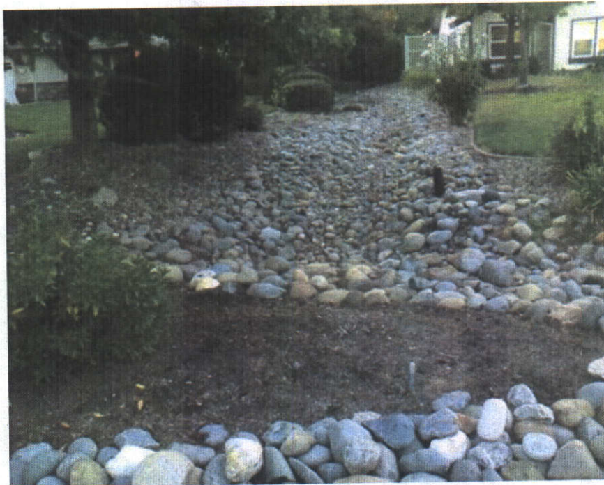
Photograph of swale taken of west side of E. Hidden Lakes Drive.
