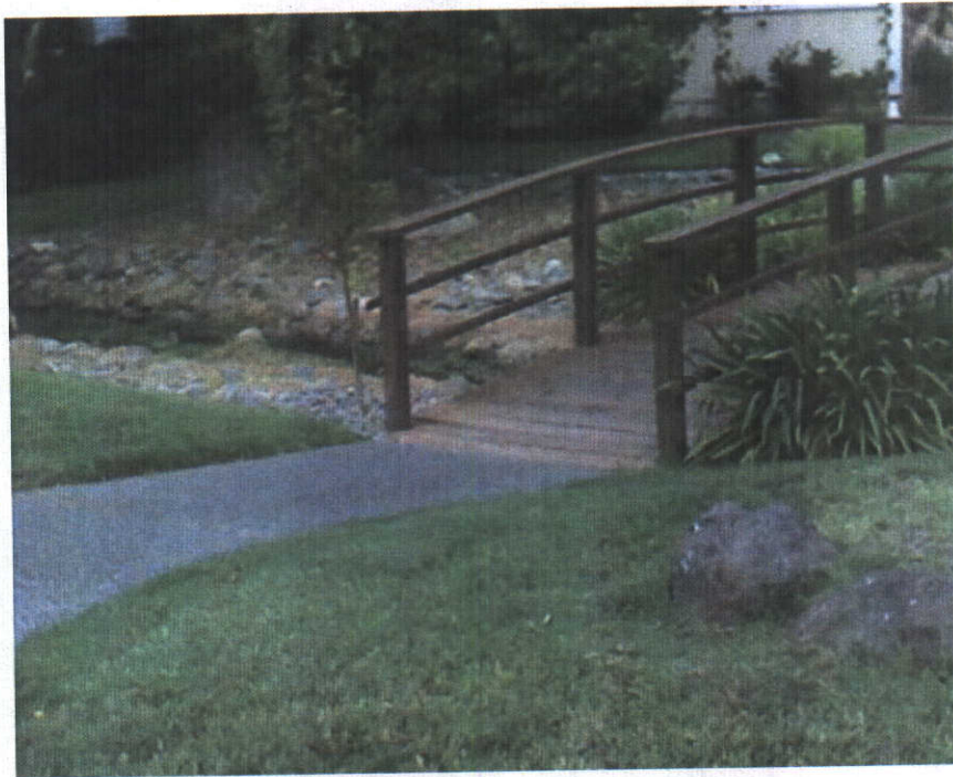
Photograph of swale taken of east side of E. Hidden Lakes Drive.
