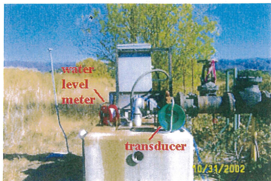
Well P6 – Well is pumping
