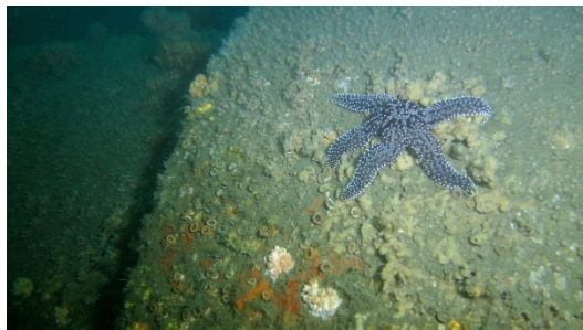
Sea Star on the Outfall Pipe
