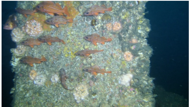
Fish at the Outfall Pipe
