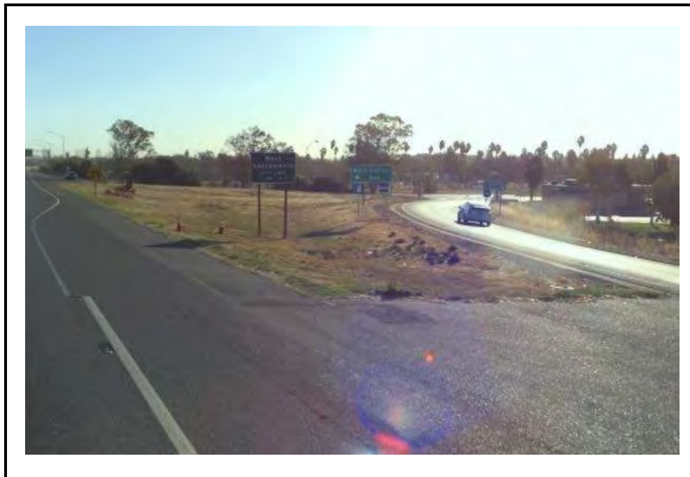
PHOTO D: VEGETATED STRIP, SWALE AND SHOULDER (NORTHWEST)
