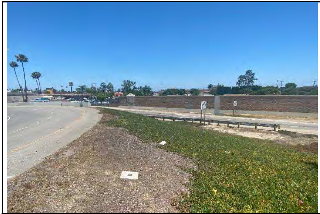
PHOTO C: Fill section with roadside vegetation strip slope flatter than 4:1 (sheet flow, 10'-20' to ditch) (NORTH)
