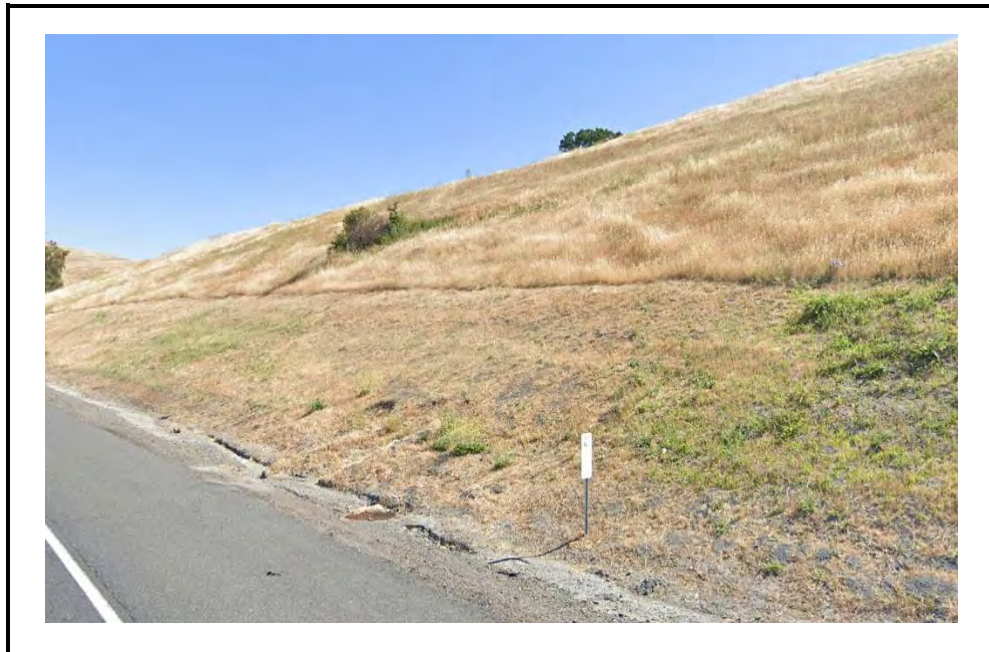
PHOTO B: CUT SLOPE, STRIP AND TRASH CAPTURE LOCATION – (NORTHEAST)
