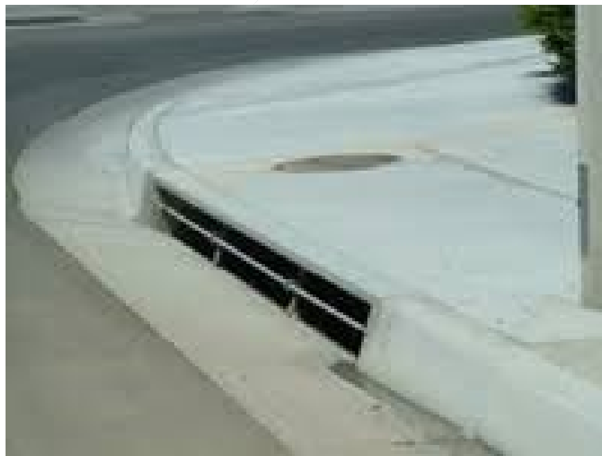
Less Common Curb Opening Inlet
