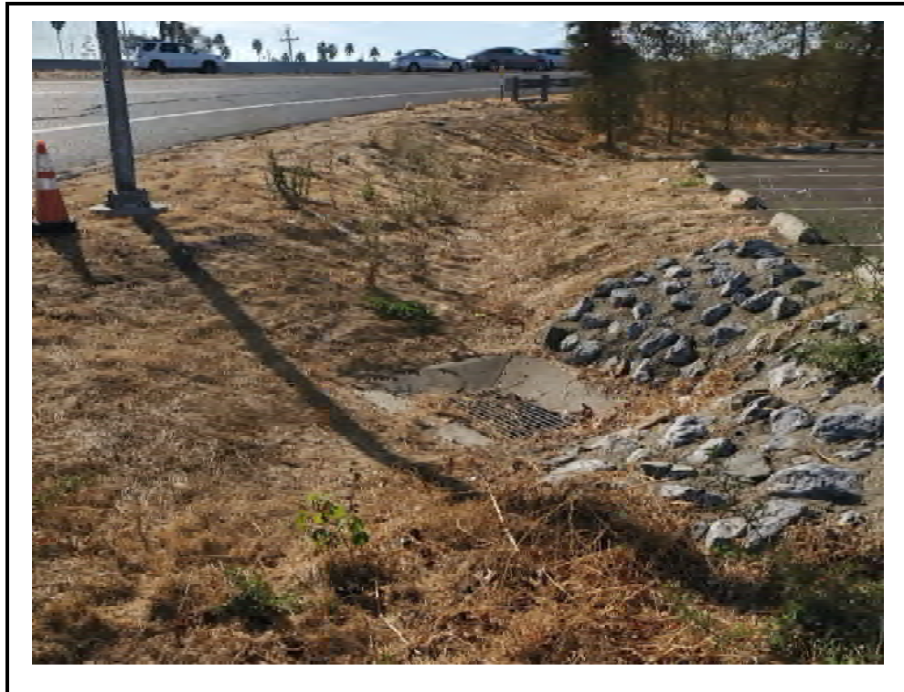
PHOTO A: DROP INLET - CAPTURE DEVICE LOCATION (SOUTH)
