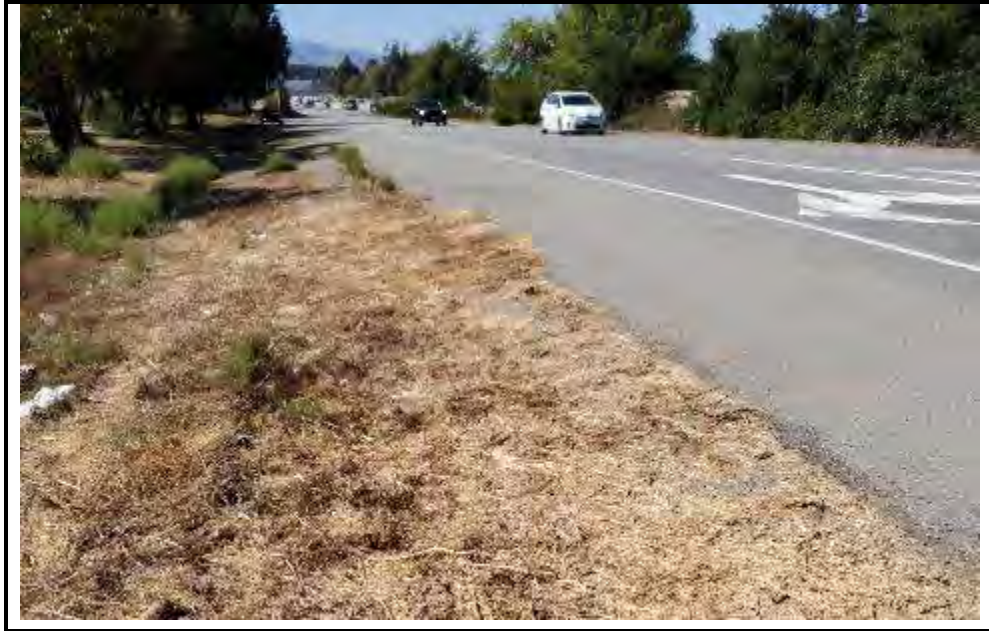
PHOTO C: VEGETATED STRIP AND SWALE (WEST)
