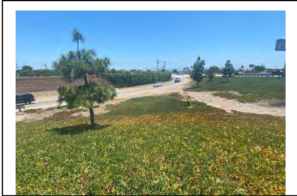
PHOTO A: Fill section with roadside vegetation strip slope flatter than 4:1 (sheet flow, 10'-20' to ditch) (WEST)
