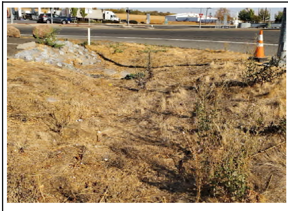
PHOTO B: VEGETATED STRIP AND SWALE (NORTHWEST)
