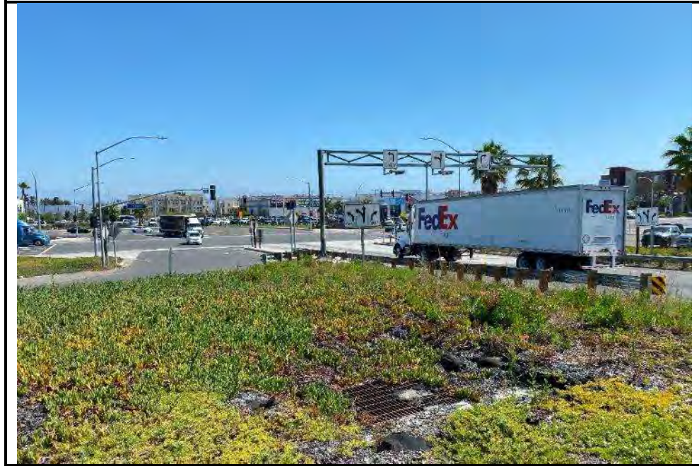
PHOTO A: Fill section with roadside vegetation strip slope between 2:1 and 4:1 (diked/curbed, 5-10' to ditch) (NORTHEAST)
