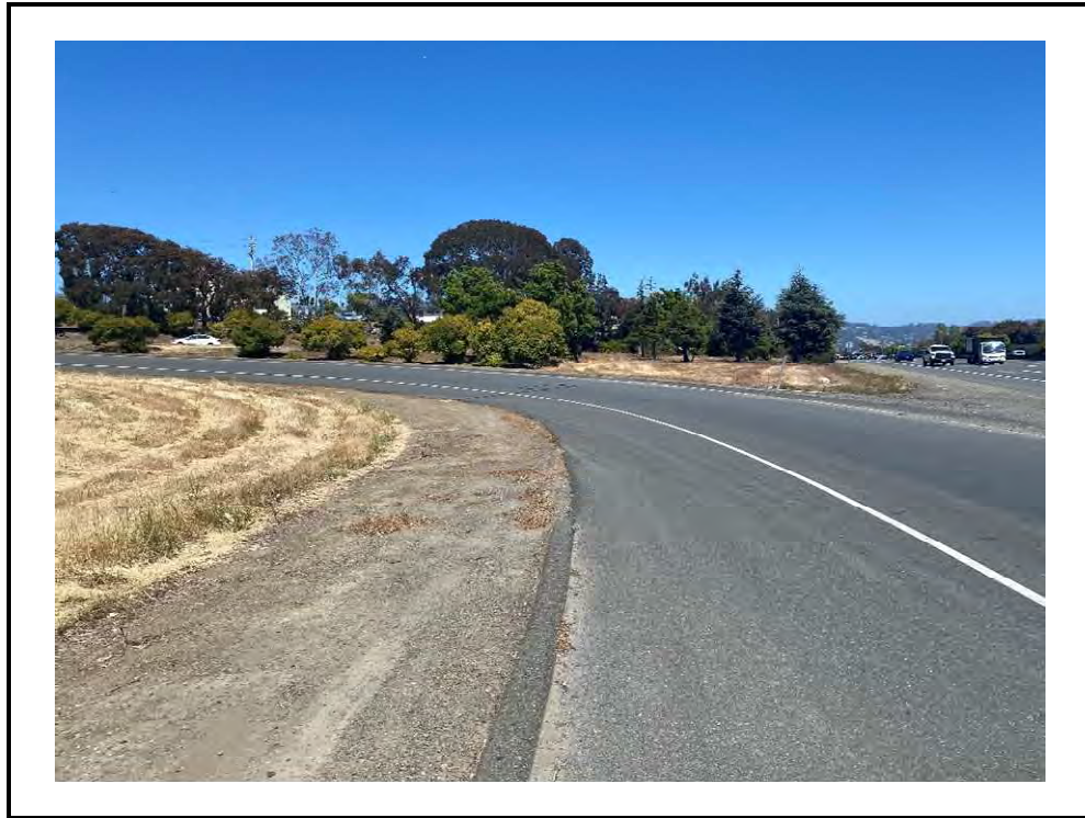
PHOTO A: CURB/DIKE – UPSTREAM (NORTHEAST)
