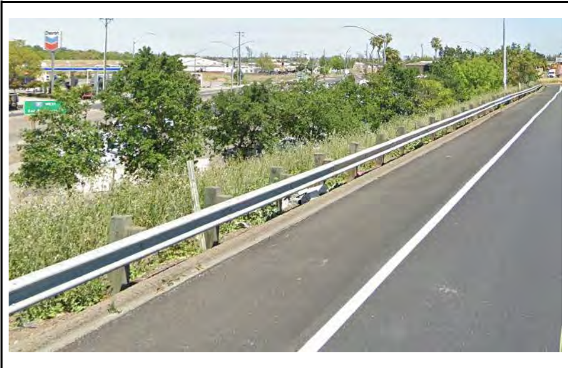
PHOTO D: ROAD AND CURB - LOOKING DOWNSTREAM (NORTHEAST)
