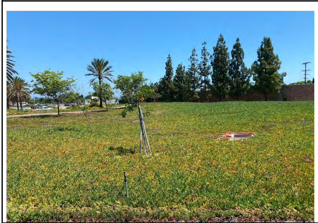
PHOTO C: Fill section with roadside vegetation strip slope flatter than 4:1 (diked/curbed, 10'-20" to ditch) (NORTHWEST)
