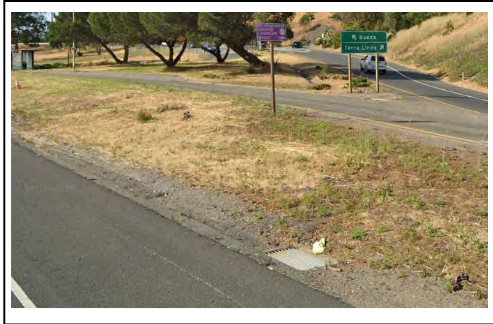
PHOTO C: DISCHARGE SUMP LOCATION (ARIAL)
