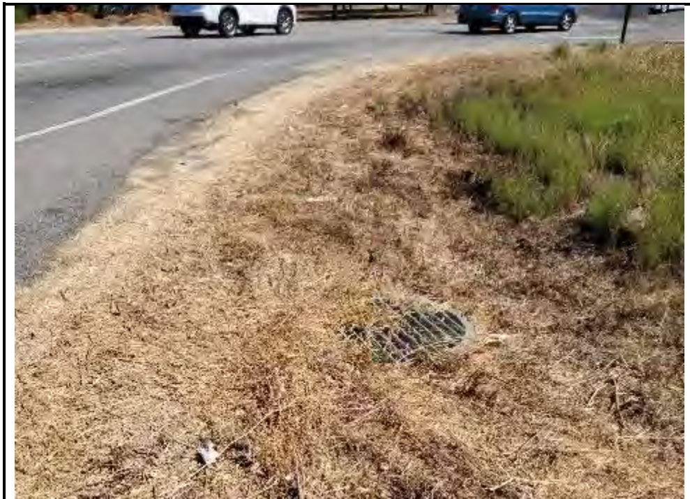
PHOTO D: VEGETATED STRIP AND SWALE AT DISCHARGE POINT (EAST)
