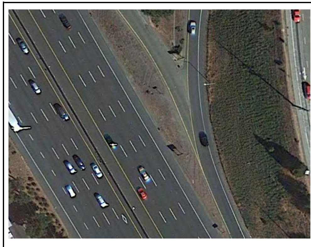
PHOTO D: DISCHARGE LOCATION (ARIAL)
