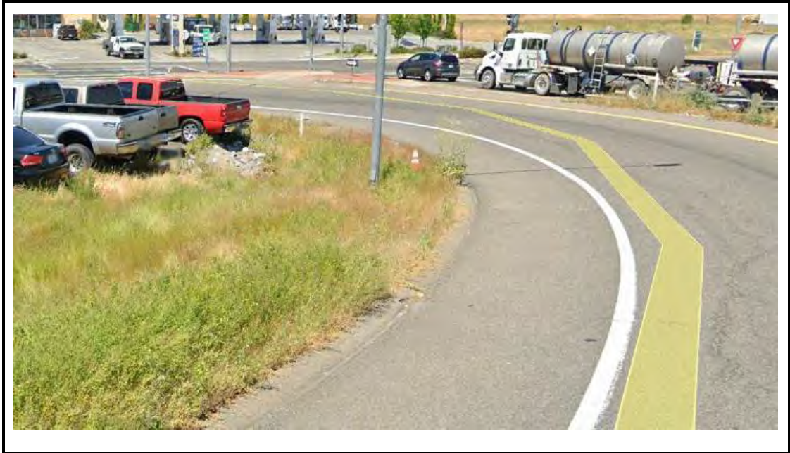
PHOTO C: ROAD, VEGETATED STRIP AND CURB - LOOKING DOWNSTREAM (NORTH)
