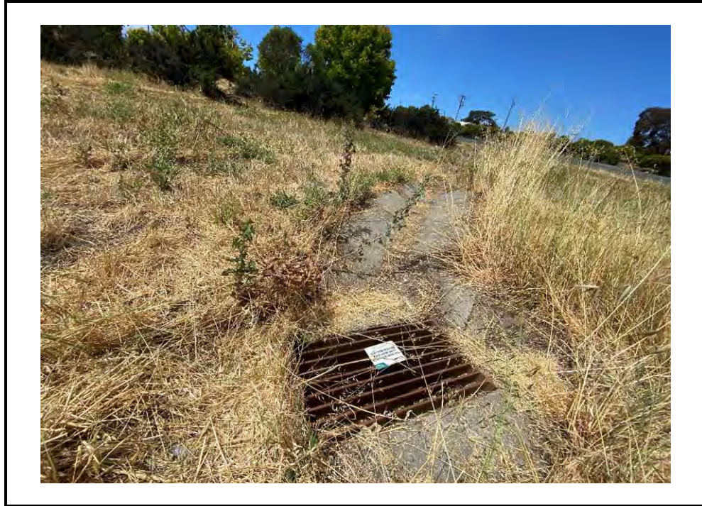
PHOTO C: VEGETATED STRIP, SWALE AND DISCHARGE POINT LOOKING UPSTREAM (NORTHEAST)
