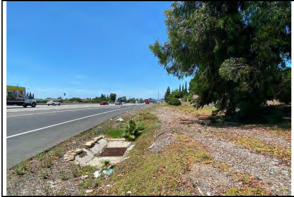
PHOTO C: Fill section with roadside vegetation strip slope flatter than 4:1 (sheet flow, 5'-10' to ditch) (NORTH)
