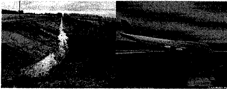
Installing or preserving open drainage channels on airports are emphasized by stormwater regulators when reviewing airfield projects. Natural or open channels are often not compatible with the airfield or FAA regulations.
