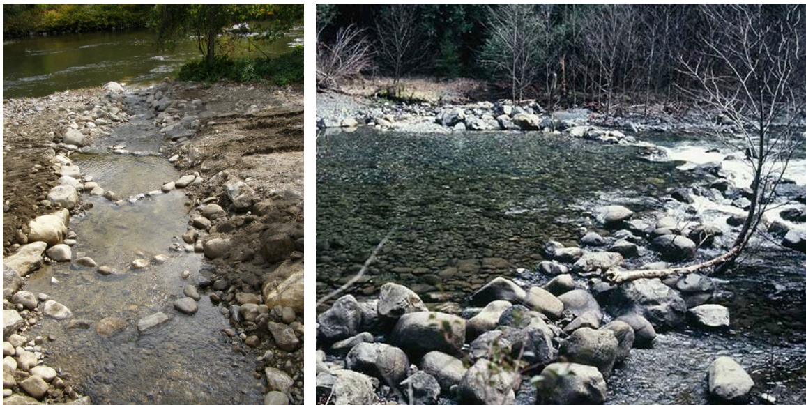
Figure 2. Examples of local cobble used to constrict flow and provide improved fish passage conditions in both small and moderate sized streams. Left picture: Spruce Brook, Connecticut, Department of Energy and Environmental Protection. Right picture: Hurdygurdy Creek, California, USDA.
