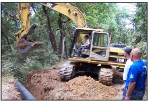
Workers install a properly sized culvert to capture water emanating from steep slopes above this rural road and direct it to a location protected from erosion.
