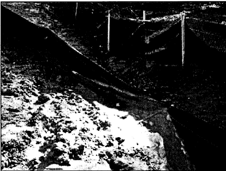
This Page: Silt fences in need of maintenance and/or replacement in various areas of site.
