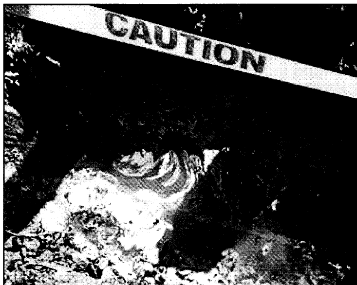
Left and Above: Dewatering (of planter area of clubhouse parking lot) was occurring when staff arrived at the site. Staff is concerned about site dewatering procedures, as person dewatering did not employ any dewatering best management practices, and did not monitor the discharge point before leaving the area. However, when staff observed the discharge point, it appeared water had not yet bypassed sandbags at the parking lot low point.
