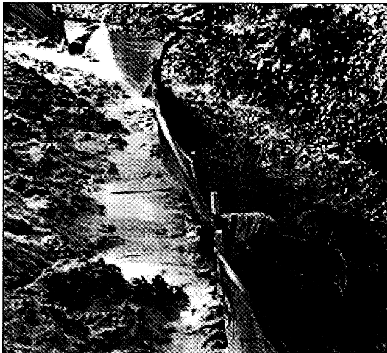
This Page: Pipes through and under silt fences in various locations on site. Such a design does not filter the runoff flowing through pipes, and results in sediment discharge.
