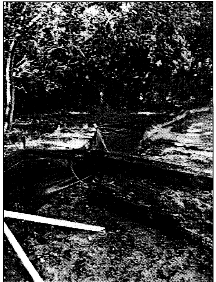
This Page: Silt fences in need of maintenance and/or replacement in various areas of site.
