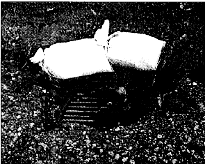
Below and Below Right: Unprotected storm drain inlets.
