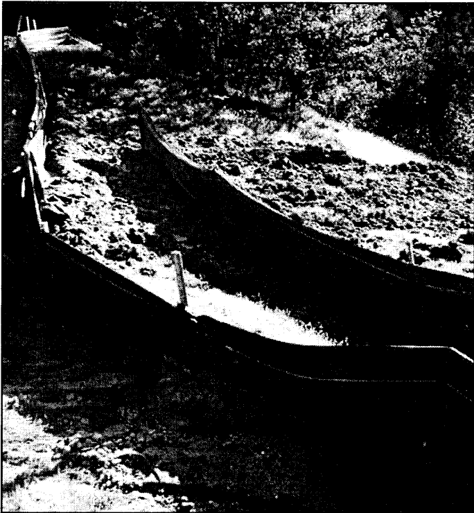
Above: Greens Complex 5. Sediment on both sides of silt fences (third silt fence to right is not visible in above photo).
