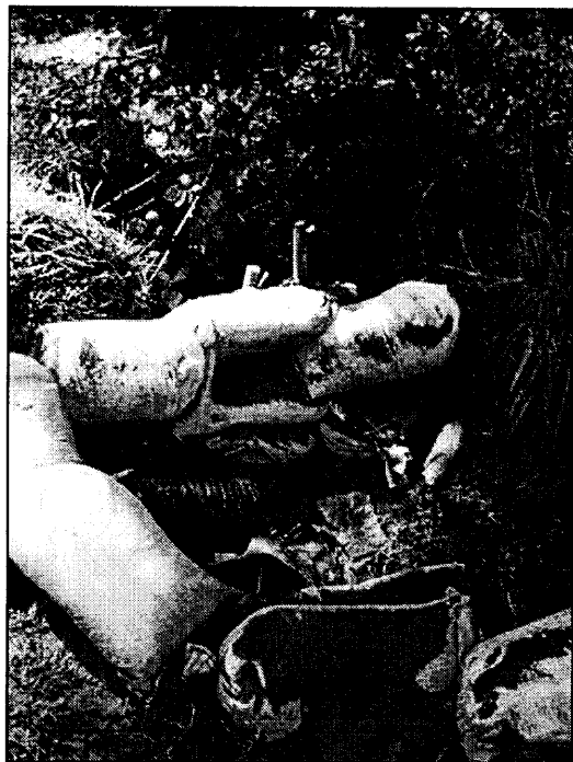
Above: Greens Complex 5. Pipes convey runoff between sandbags.
