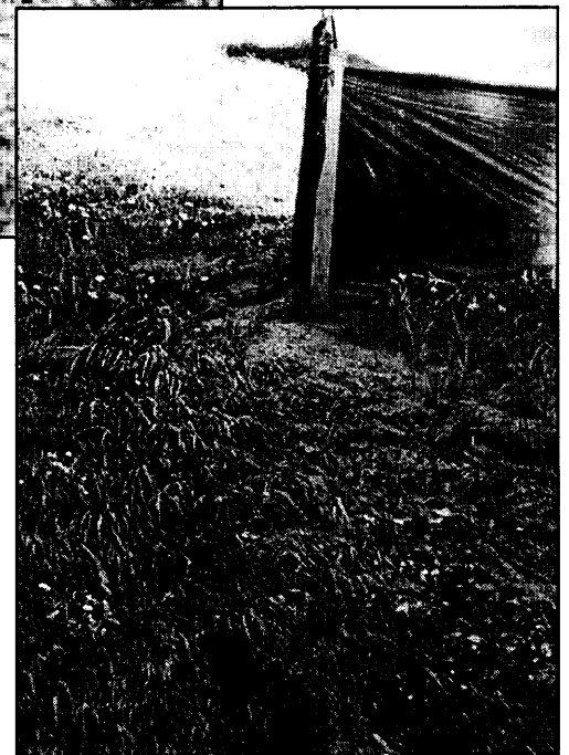
Top Right: pipe on other side of fence. Sediment in grass is evidence of muddy water discharge from pipe.
