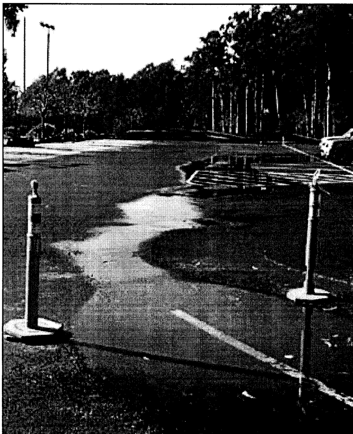
Left and Above: Dewatering (of planter area of clubhouse parking lot) was occurring when staff arrived at the site. Staff is concerned about site dewatering procedures, as person dewatering did not employ any dewatering best management practices, and did not monitor the discharge point before leaving the area. However, when staff observed the discharge point, it appeared water had not yet bypassed sandbags at the parking lot low point.
