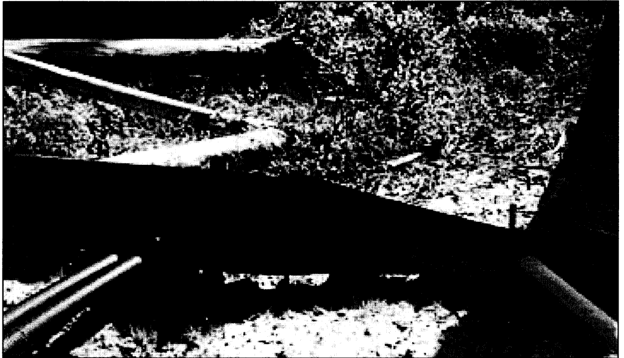
This Page: Pipes through and under silt fences in various locations on site. Such a design does not filter the runoff flowing through pipes, and results in sediment discharge.
