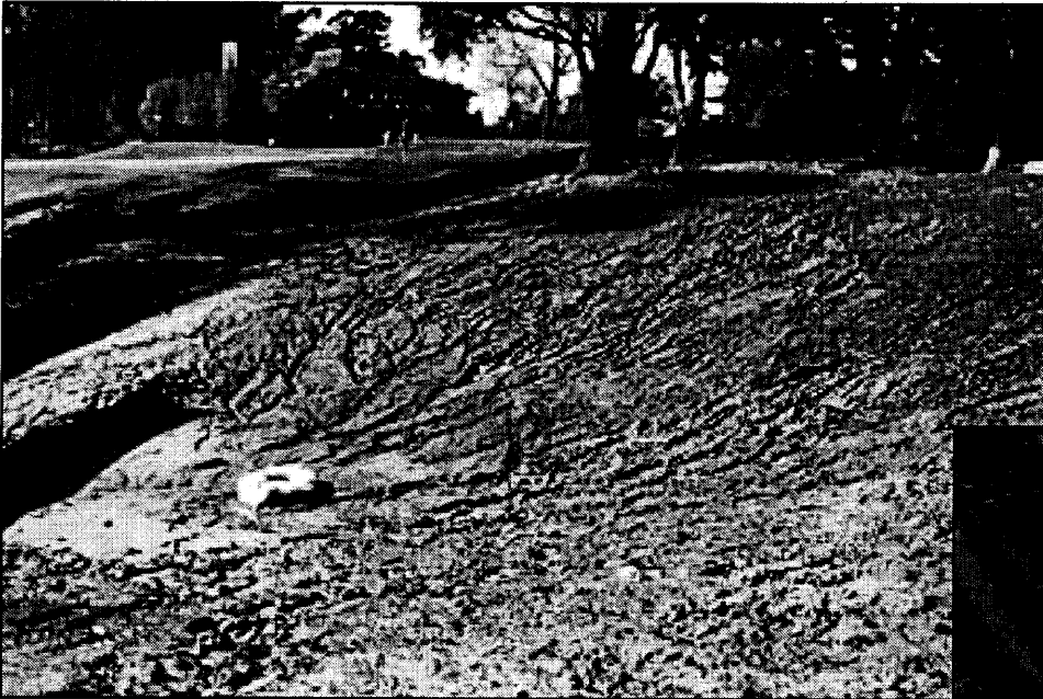
Above and Right: Greens Complex 18 drainage inlet protection added since last inspection. However there is still significant erosion on slopes (above) and a hole in the filter fabric (right).
