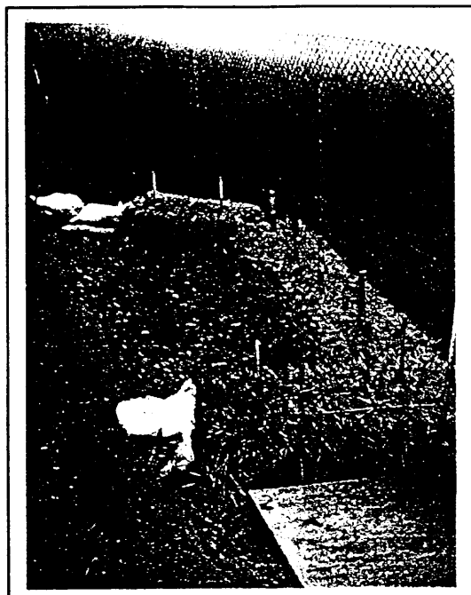
Photo 3 – Sediment trap for southern discharge location.
